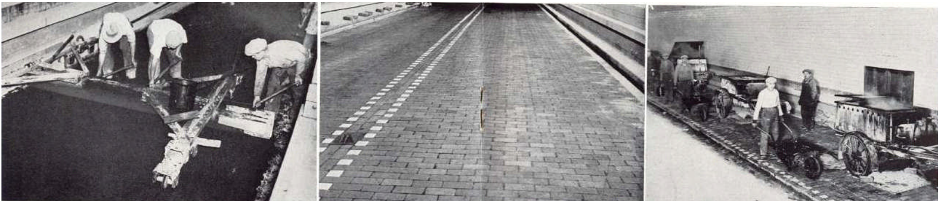
Above Left-to-Right: caption: “Striking off asphaltic-sand mastic bed course with screed traveling on rollers and discs with compensating carriage / Close-up view of completed brick pavement showing clean wire-cut skid-resistant traffic surface / Kerosene fueled heating kettles in which ‘blended’ asphalt filler was heated to 450-degrees F”
