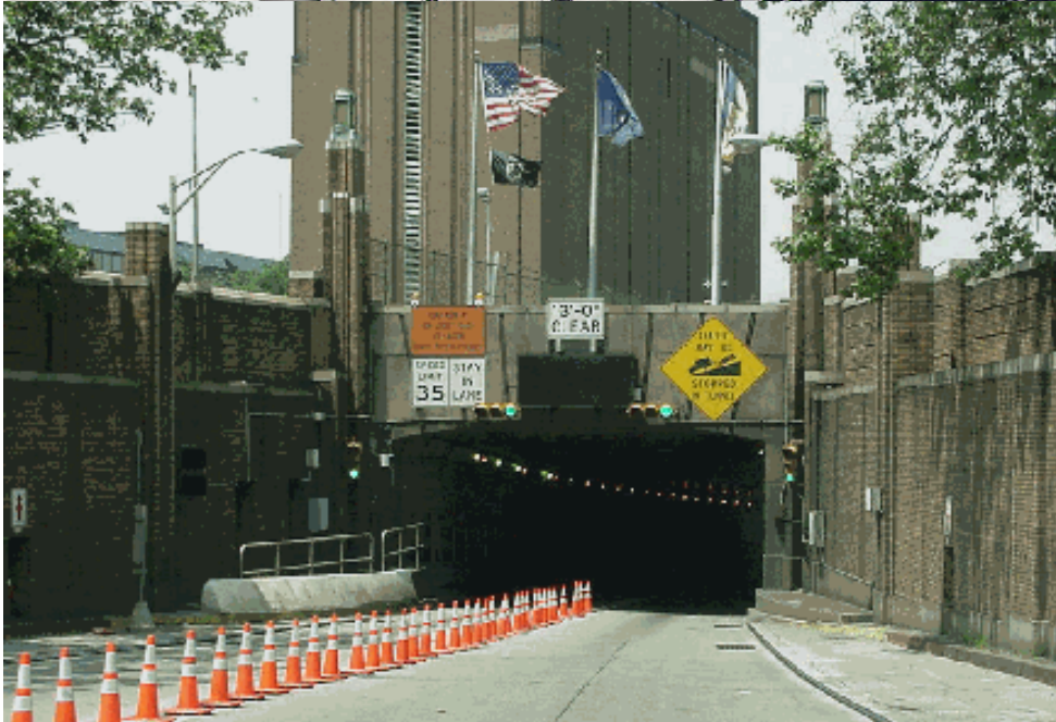
Bottom: caption: “Photo shows the Art Deco-style Manhattan portal of the Lincoln Tunnel and the east ventilation tower”
