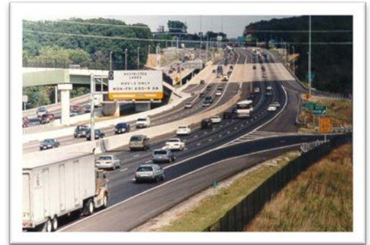
Figure 1-2: HOV Lane on Interstate 95 in Woodbridge, VA
