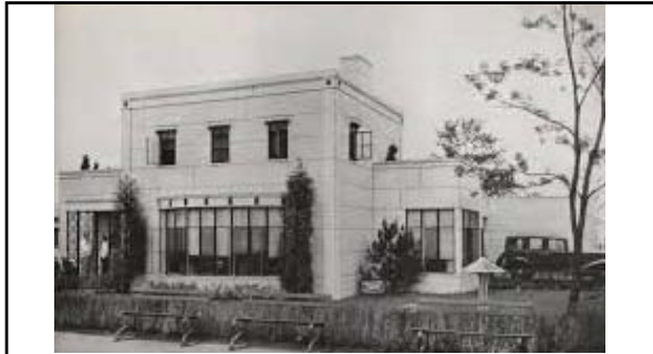
Above: to provide a fireproof surface for the outer covering of the Good House-keeping-Stran-Steel House , eight-by-two foot sheets of three-inch thick baked-iron enamel were used to cover the outside. The baked surface of the material gave the illusion of brick and helped to insulate the house. 229
