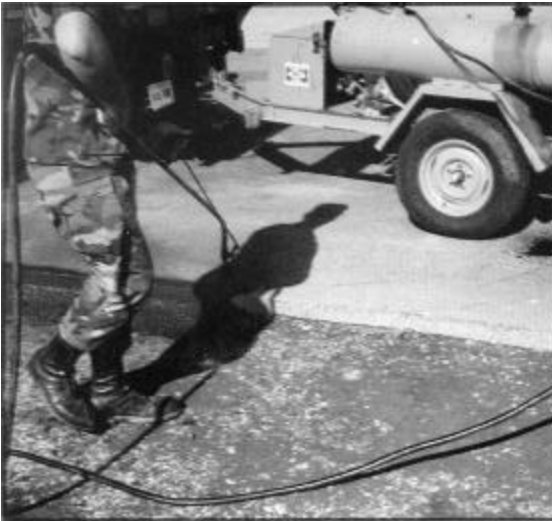
Figure 3.7. Applying tack coat with spray wand
