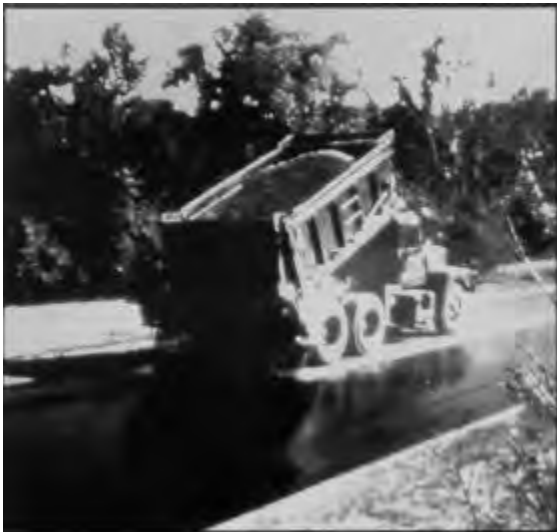
Figure 5.1. Applying aggregate with tailgate spreader on dump truck
