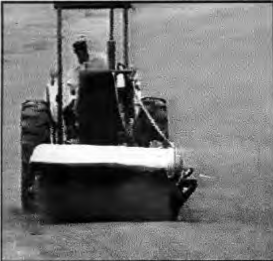
Figure 5.3. Brooming the treated area
