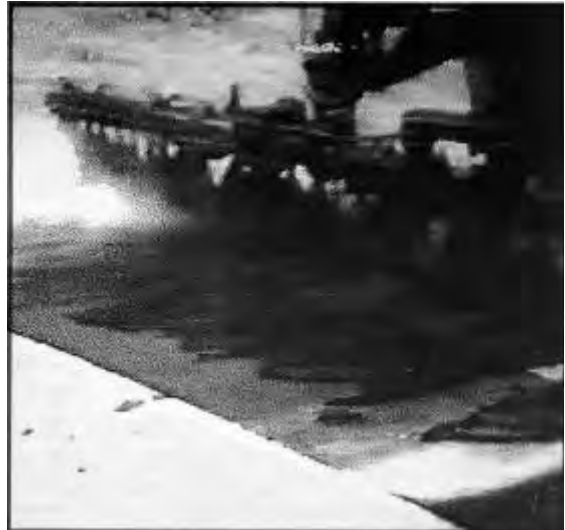
Figure 5.4. Straight edge formed after building paper removed
