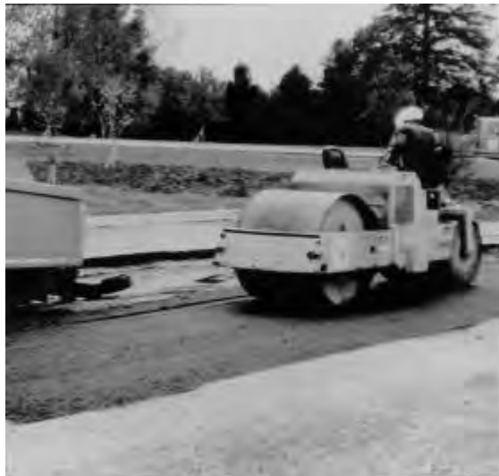
Figure 3.10. Steel-wheel roller
