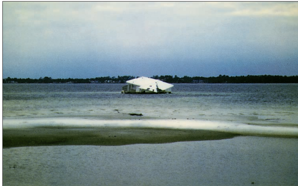
Figure 1-9. During Hurricane Opal (1995), this house was in an area of channeled flow between large buildings. As a result, the house was undermined and washed into the bay behind a barrier island.
