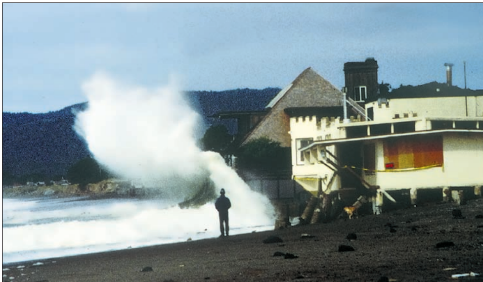
Figure 1-10. Storm waves breaking against a seawall in front of a coastal residence at Stinson Beach, California.
