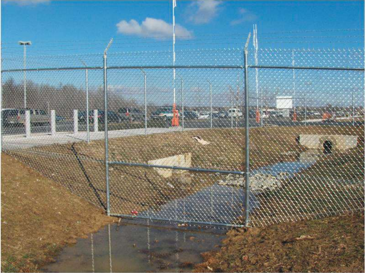
Figure 19 Chain link fence over ditch
