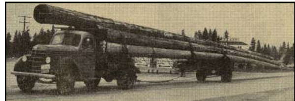
Above: caption: "When Consolidated Builders, Inc. wanted some big poles for raising mixing plant lines at Coulee dam, it was up to B.J. Carney Company, Spokane, to deliver the goods. The picture shows one of their trucks loaded with six 90-foot poles en route to the dam. These overgrown toothpicks presented many problems in handling, as their length of 90-feet and their weight of 22,000 pounds provided man a traffic hazard. A special license to have them on the highways, a pilot, and a police escort to turn corners on their way through the city were just three of the many angles that had to be worked out in advance. The trees were logged and trucked from the Priest River area." (Spokane Chronicle, April 16 th 1938)
