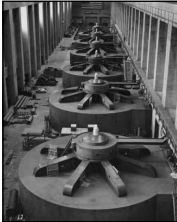
Popular Mechanics, May 1942 Left: caption: "Interior of Grand Coulee Dam power plant showing six of nine generators in-place, ca, 1940) 1573
