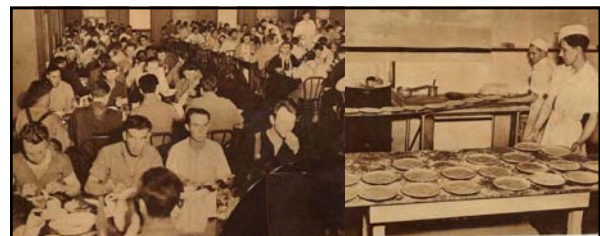
Left: caption: "Because of the many shifts building Grand Coulee Dam, almost continuous service is maintained in the mess hall. Here is a view of one of the wings in the main dining room, seating 512 persons. Another seats 288. One thousand Sunday visitors often share tables with the 5,000 dam builders." ( Seattle Times , May 30 th 1937) Right: caption: "Feeding Coulee Dam's 5,000. A board holding eleven pies is shoved in the oven while Soren Juul prepares more. Nice cases of fruit (apricot at this baking) fill the 438 pies needed for one meal. When the oven is loaded there are seventy-three pies baking." 1002 ( Seattle Times , May 30 th 1937)
