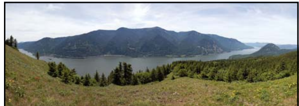
"...The gorge of the Columbia river is too big to permit an arch-type dam. Grand Coulee must depend upon its massive weight alone to resist the pressure of the water it will back up. At the dam site the river is 700-feet wide and at times seventy-feet deep, flowing fourteen miles an hour, and has an annual average runoff of 79,000,000 acre-feet, five times that of the Colorado at Boulder dam..." Popular Mechanics, April 1938
