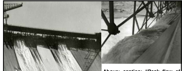
Above: caption: "Peak flow of the annual flood stage of the Columbia River is discharged over the dam in special diversion channels. 05/29/1940." Left: caption: "Cascading Columbia River flood waters pour through the spillway diversion channels in waterfalls higher than Niagara. 5/27/1940." 1418
