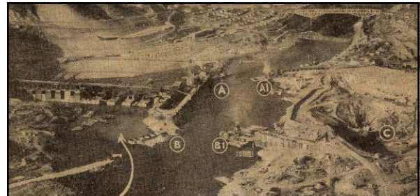
Above: caption: "The picture shows what the reclamation association delegates saw during their Sunday visit. The aerial picture was taken Saturday, looking downstream. It is the first taken since the diversion was started. The arrow indicates the new course of the river, through openings in the dam foundation. The letters A, A-1, B and B-1 indicate where coffer dams are being constructed across the river channel. Between these coffer dams, the engineers will build the dam proper. The east shore cofferdam is shown on the right, holding the river out from the area marked C, where concrete for the east abutment will soon be poured." ( Spokane Chronicle, June 1936 )
