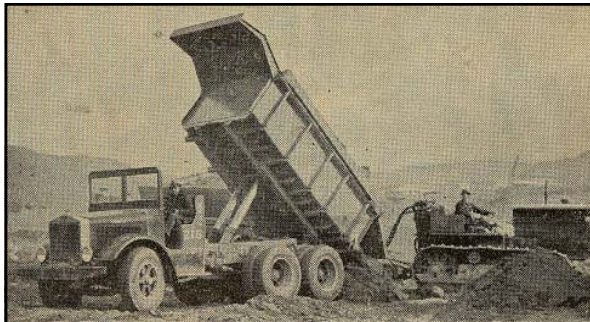
Above: caption: "Among the latest deliveries of large trucking units is a fleet of six whites with specially built bodies to carry 12 cubic yards of material, to MWAK. One of the fleet is shown in the picture. The body was built by the Union Iron Works here, chassis being furnished through the White factory agency. The job has six wheels with two tires on each of the four rear wheels. There are two drive axles, making possible pulling through soft material much as a caterpillar tractor pulls through mud and soft spots. The picture shows one of the units unloading material on the 'grizzly' which screens out the rocks, preventing injury to the machinery handling the dirt. Gross load of the unit in operation is 60,000 pounds." 1185 ( Spokane Chronicle , March 20 th 1935)
