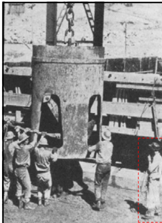
"...As the dam grows, in 5-foot 'lifts,' placed in any column at intervals of not less than 72 hours, the steel trestles are buried, and forever lost..."
