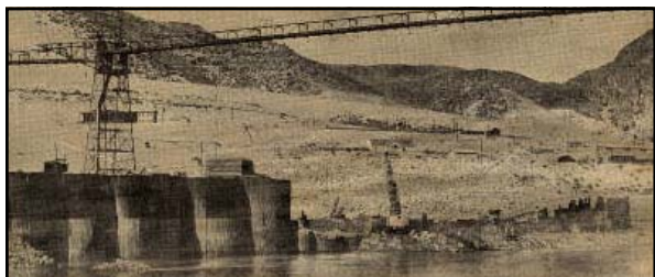
Above: caption: "Make way for the Columbia! That is what MWAK workmen are doing in west shore operations at the Grand Coulee dam project, where, within six or eight weeks, the mighty Columbia will be diverted about 200-feet from its original channel. In the right portion of the picture, destruction appears to have struck the steel cofferdam. However, such is not the case as the cofferdam is being removed at this point to make a passageway for the river after it flows over the west shore concrete dam foundation. The height at which the Columbia will travel through its new channel is shown by the high water line on the cluster of steel cofferdam in the left of the photograph. The high water line is about 50-feet above the present low water level. The downstream face of the diversion 'crib dam' will tie into the steel cofferdam at the extreme left end where the tall sheet pilings still are standing." (Spokane Chronicle, September 23 rd 1936)
