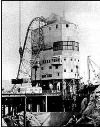
“...Concrete is mixed in two plants, octagonal tower-like structures 44-foot wide and more than 100-feet high, one originally located on each side of the river. At the top of each plant are two bins for cement, one for sand, and one for each of the four sizes of gravel used. By means of electrically operated devices, under push-button control by one operator, water, cement, sand, and gravel of each size, in quantities appropriate to the mix required, are automatically weighed out for each batch and delivered to one of four 4-yard mixers in each plant, graphic records of all components and the consistency of each batch being automatically recorded...” U.S. Bureau of Reclamation (ca. 1937) Left: caption: “Giant concrete factory, capable of turning out enough concrete in one month to build a two-lane highway more than 250 miles long”
