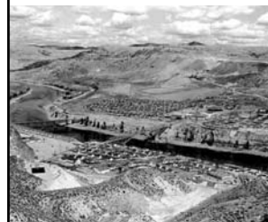
"...Getting ready to build the dam was a major job in itself. Two towns, a 'contractor's town' and a 'government town,' were built on opposite sides of the river for the nearly 6,000 workmen and engineers..."
