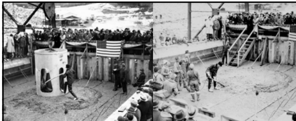
The first bucket of concrete was poured into Grand Coulee Dam by Washington State Governor Clarence D. Martin on December 6 th 1935 while a large crowd gathered for the event looked on. After this initial pour, only 2,624,000 bucketsful of concrete remained to be poured. Each bucketful added four cubic-yards (eight tons) to the concrete mass of the dam.
