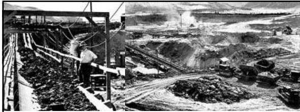
"...For several months the MWAK Company has been using more than three miles of conveyor belt in the removal of the overburden from the dam site to Rattlesnake canyon, which today holds more than 12,000,000 yards of gravel and clay. Rattlesnake canyon, once a gorge several hundred feet deep, now is filled practically level with the surrounding country..."
