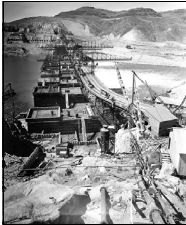
"Heading down the home stretch, the MWAK Company started on its last million yards of concrete Sunday...It has taken the company almost two years to pour the 3,500,000 yards, or about 1,750,000 a year. It is predicted, with the company having averaged more than 100,000 in a single week, that the remaining 'mud' will be placed in little more than 10 weeks. Even during the pouring of the first 3,500,000, MWAK shattered every type of world record. More than 15,700 yards were placed in a single day, which is 5,000 yards more than recorded in a day at Boulder..." Spokane Chronicle, September 6 th 1937 1459
