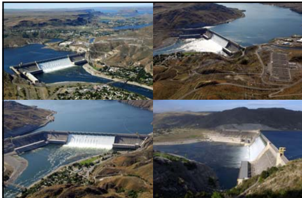
Above: caption: "June 30, 2011. Aerial view of Grand Coulee Dam releasing downstream an unusually large and late spring time water flows of over 200,000 cfs. Broken out, it's 33,800 cfs, over the spillway and 167,000 cfs through the hydropower generators." 1653
