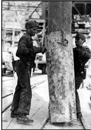
"Some of the romance of the old days has come back to glorify the cause of common labor. It has come to attention at Coulee dam, where a crew of men poured 8,400 cubic yards of concrete in one day, before work was shut down, to set a national record. This kind of work, reminiscent of the spirit of competition which made a picturesque page of construction history in the early part of the century, is a gratifying indication that men again are taking pride in achievement. These men might have 'strung out their jobs' by slow work which would have extended the time of construction. But they are made of the stuff Americans like to have in their being. This comes at a time when too many men, their spirit broken by being dependent, feel that the world now owes them a living. During the last week 1,000 men have added to the MWAK payroll. Work soon will be humming again at high pitch. Other records will be assailed. Americans, living in a land of opportunity for the individual, will do work which is a credit to the name 'American.'" 913 Spokane Chronicle, March 12 th 1937
