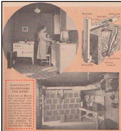
Left: caption: "Electricity Transforms The Home. A kitchen at Mason City, equipped with all electrical conveniences. The drawing shows construction of experimental heat-storage oven to use off-peak current loads for heating in winter. At right, an oven installed for trial in a house at the dam-site village."
