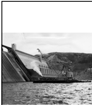
Left: caption: "Despite the absence of flow down Grand Coulee dam's spillway, the Columbia river is choppy as a huge barge with its steam-operated crane dredges out debris. Turbulence is caused by underwater pressures from the powerhouse out-pourings. The dredge, which first saw service in 1949-51 after the 1948 flood, will be operated on a two-shift-per-day basis five days a week until high water this summer forces the operation to cease. The dredge moves downstream periodically so that discharge tubes can spill water from Lake Roosevelt, whose level has remained high all winter."
