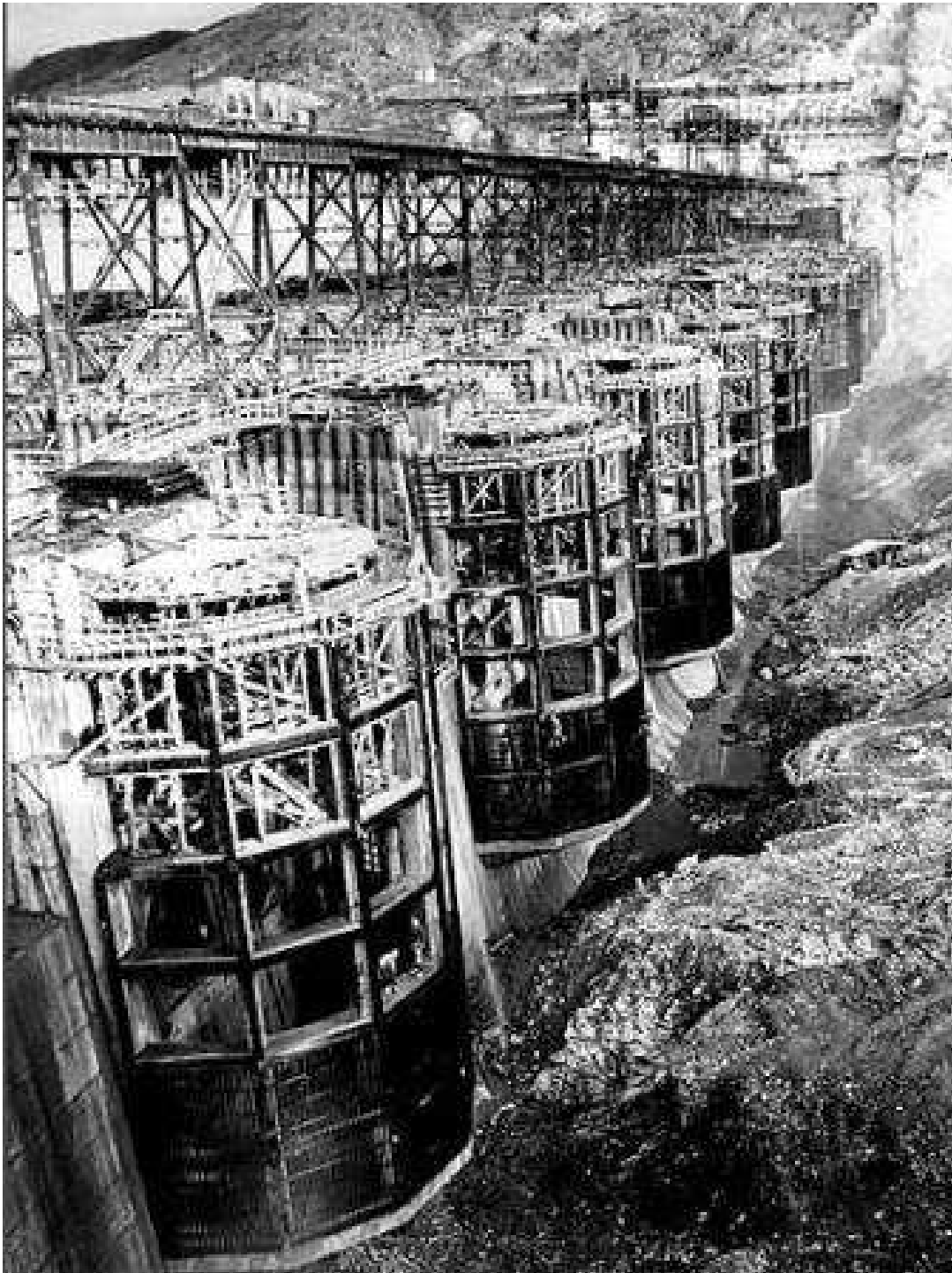
Above & Left: caption: “Trash racks on the upstream face of the dam built to protect outlet tunnels from debris, Grand Coulee Dam construction, November 1937”
