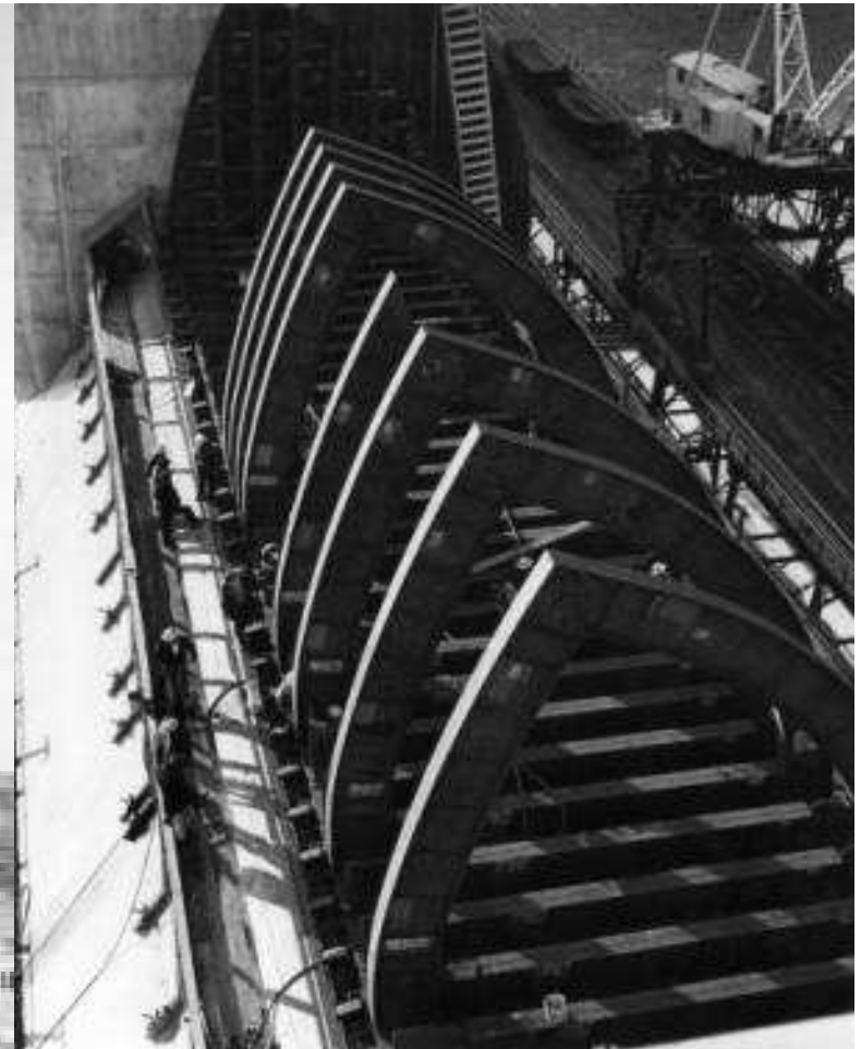
Above: caption: “Installation of main girders for drum gate Number One, December 1940”
