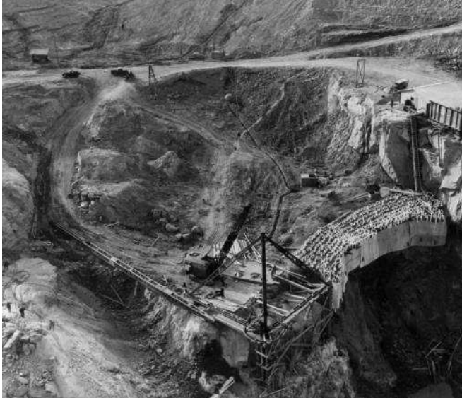
Top Left: caption: “A 5-yard electric shovel and 10-yard buggies working in the diversion channel, August 1936”
