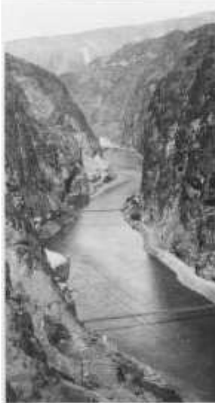
COMMENCEMENT OF CONSTRUCTION 1931
