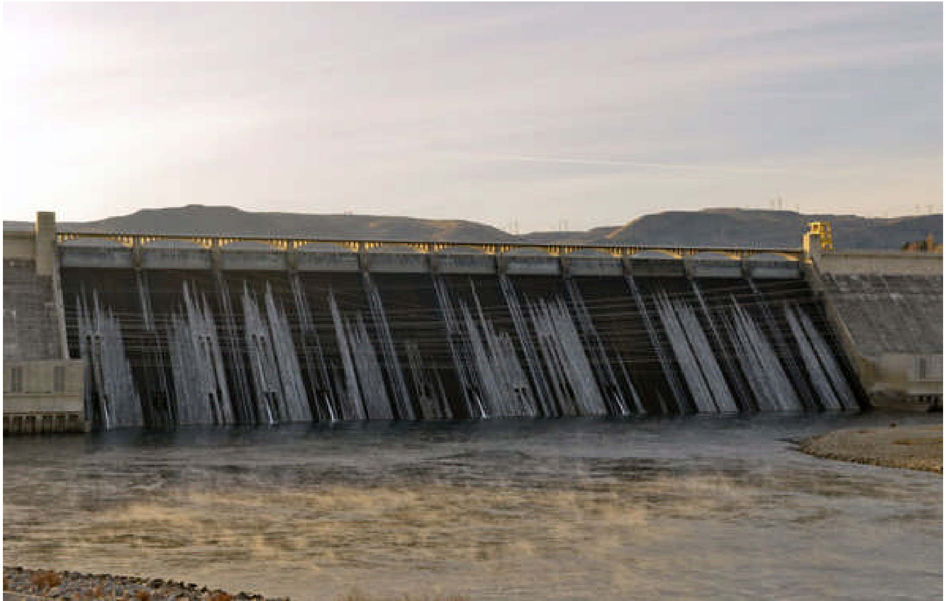
Above: caption: “November 2013. Grand Coulee Dam in the morning light. The cold November air causes water to freeze on the face of the dam and steam to rise from the water in the stilling basin.”
