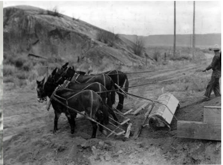
Above: caption: “Preparing bed with mules for laying ties for the railroad spur from Coulee City to Grand Coulee Dam (ca. 1935)” Left: caption: “Supply Train. Coulee City - Coulee Dam Railroad”
