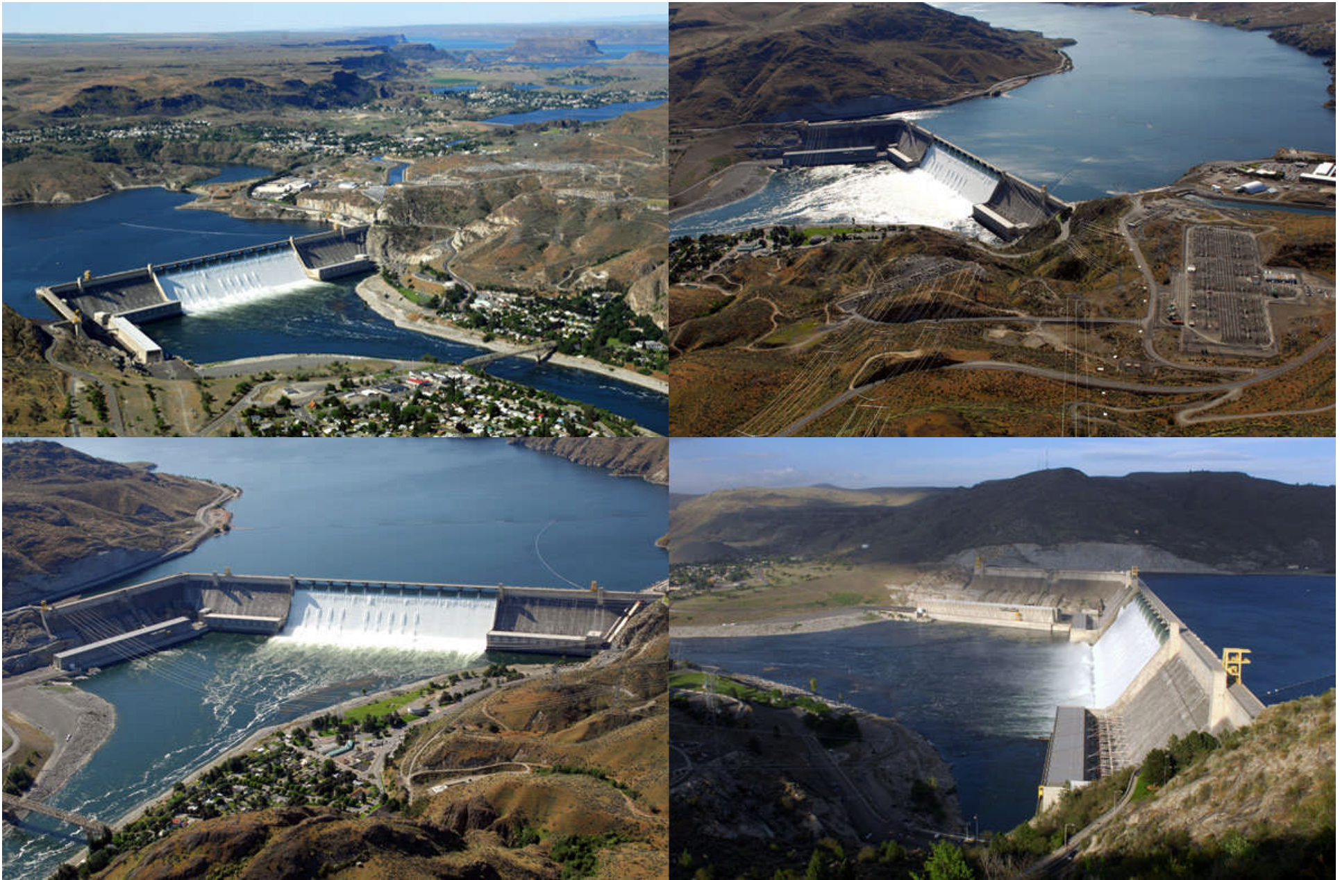
Above: caption: “June 30, 2011. Aerial view of Grand Coulee Dam releasing downstream an unusually large and late spring time water flows of over 200,000 cfs. Broken out, 1653 it’s 33,800 cfs, over the spillway and 167,000 cfs through the hydropower generators.”
