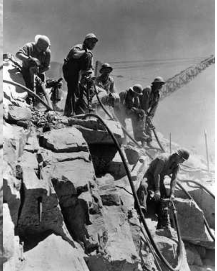
Above: caption: “Drilling blasting holes in rock face for Grand Coulee Dam (ca. 1938)”
