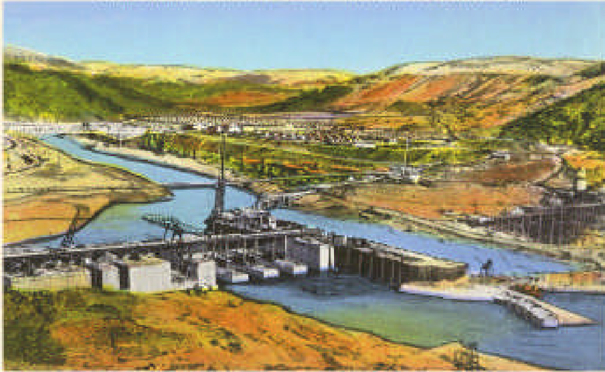
AT GRAND COULEE DAM, STATE OF WASHINGTON
