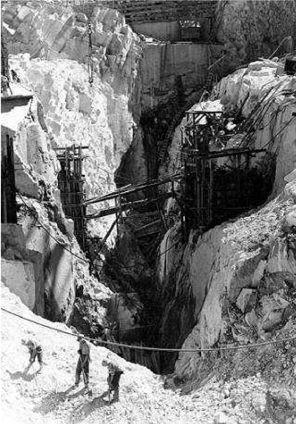
Above & Left: caption: “Workers drilling bedrock at Grand Coulee Dam site, July 1937” 1241
