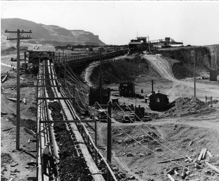
Top Left: caption: “Electric shovels and belt conveyors move 25,000 yards of pit-run sand and gravel in a day”
