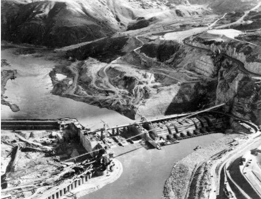
Top Left: caption: “You can see how the cofferdam clears a portion of the riverbed for excavation”
