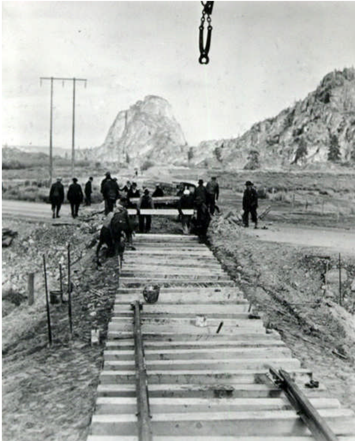
Above: caption: “Preparing bed with mules for laying ties for the railroad spur from Coulee City to Grand Coulee Dam (ca. 1935)” Left: caption: “Supply Train. Coulee City - Coulee Dam Railroad”
