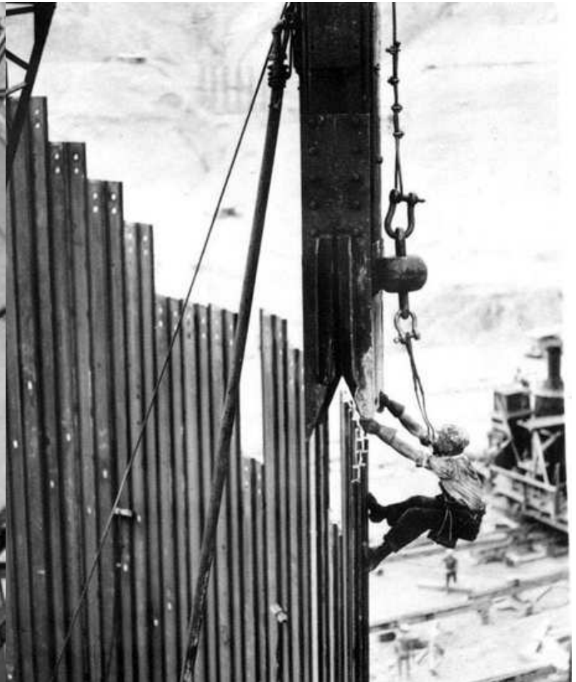
Above: caption: “Setting a 3&1/2 foot-ton steam hammer for driving piles in cofferdam connecting section ‘C’ with block 40 (August 1936)”
