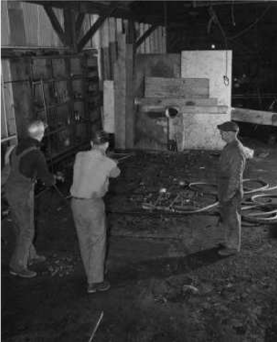
Above: caption: “Re-boring drum gate girder. Machine shop – powerhouse, January 1941”
