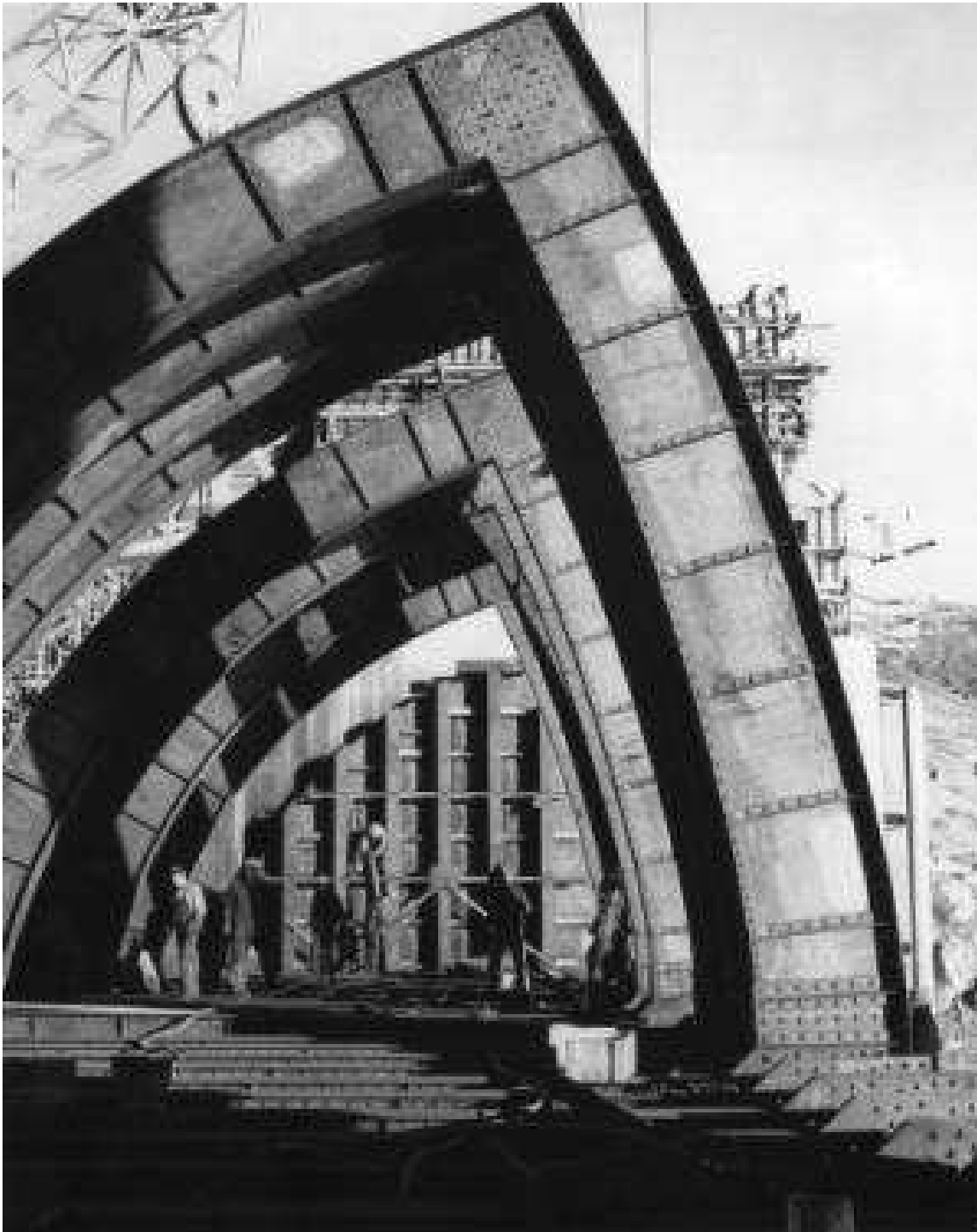
Above: caption: “Installation of main girders for drum gate Number One, December 1940”
