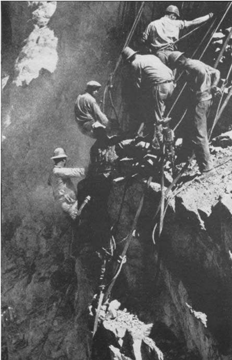
Above: caption: “Jackhammer crews drilling blasting holes at Grand Coulee Dam, 1938”
