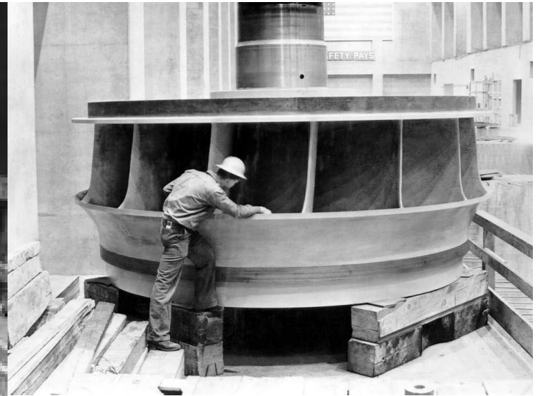
Above: caption: “Workman inspecting one of the generator turbines just before its installation. Photo was taken on December 18, 1942.”
