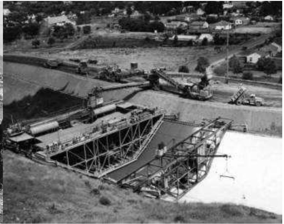
Top Left : caption: “Excavation for the feeder canal at Grand Coulee Dam (December 1946)”
