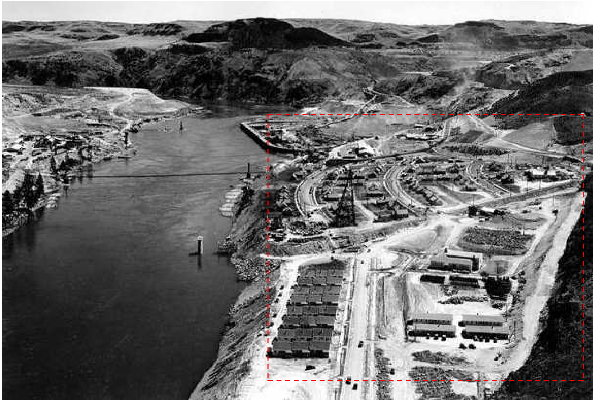
Above: caption: “Grand Coulee Dam construction site panorama, July 1935” (Engineers’ Town highlighted)
