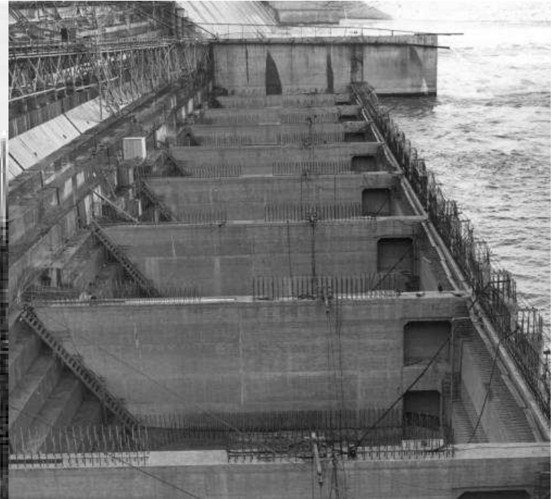
Above: caption: “General view of reinforcing steel at East Powerhouse base, October 1940”
