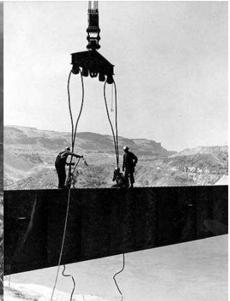
Above: caption: “Workers at Grand Coulee erect a large steel girder”
