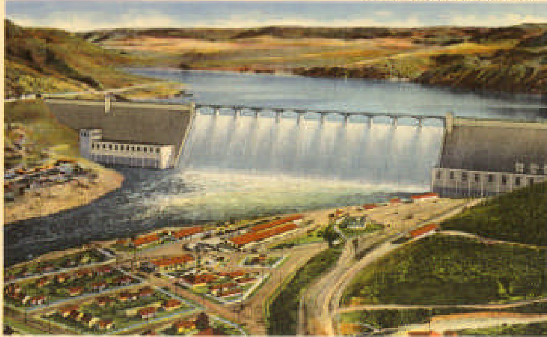
Grand Coulee Dam, Washington
