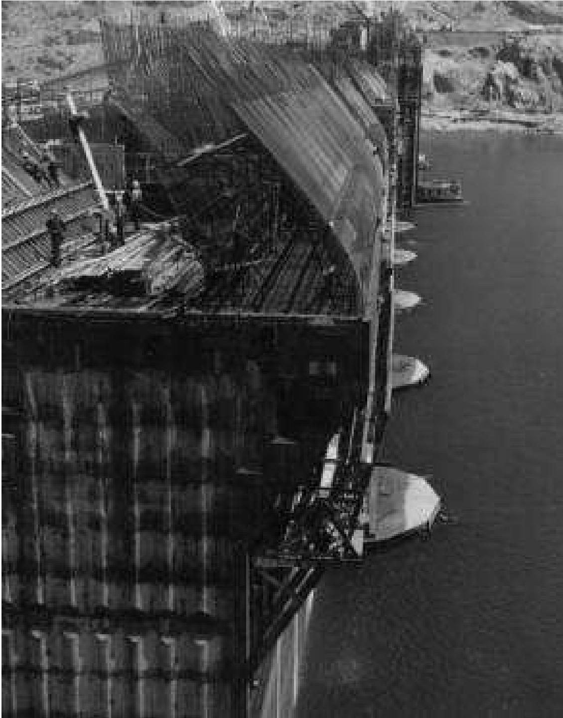
Above & Left: caption: “Steel and Form work for drum gate install- ation. Steel is for spill- way crest, bridge piers, and drum gate chamber, June 1940”
