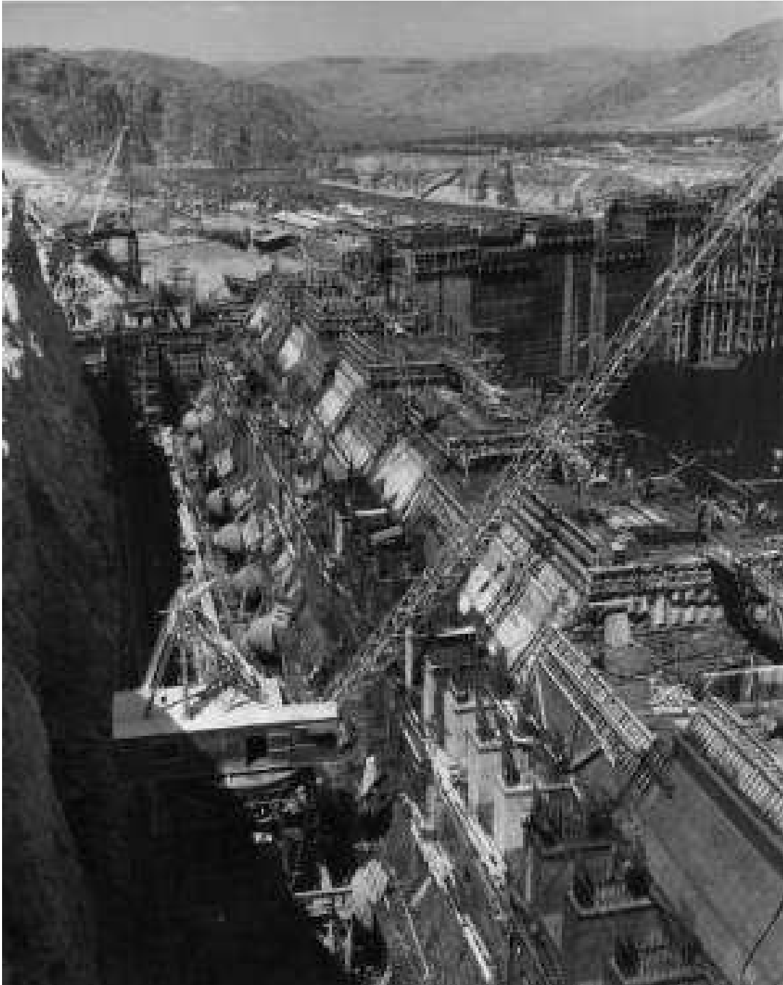
Above: caption: “Coulee Dam irrigation pumping plant and discharge pipes – west crane recess, April 1940”
