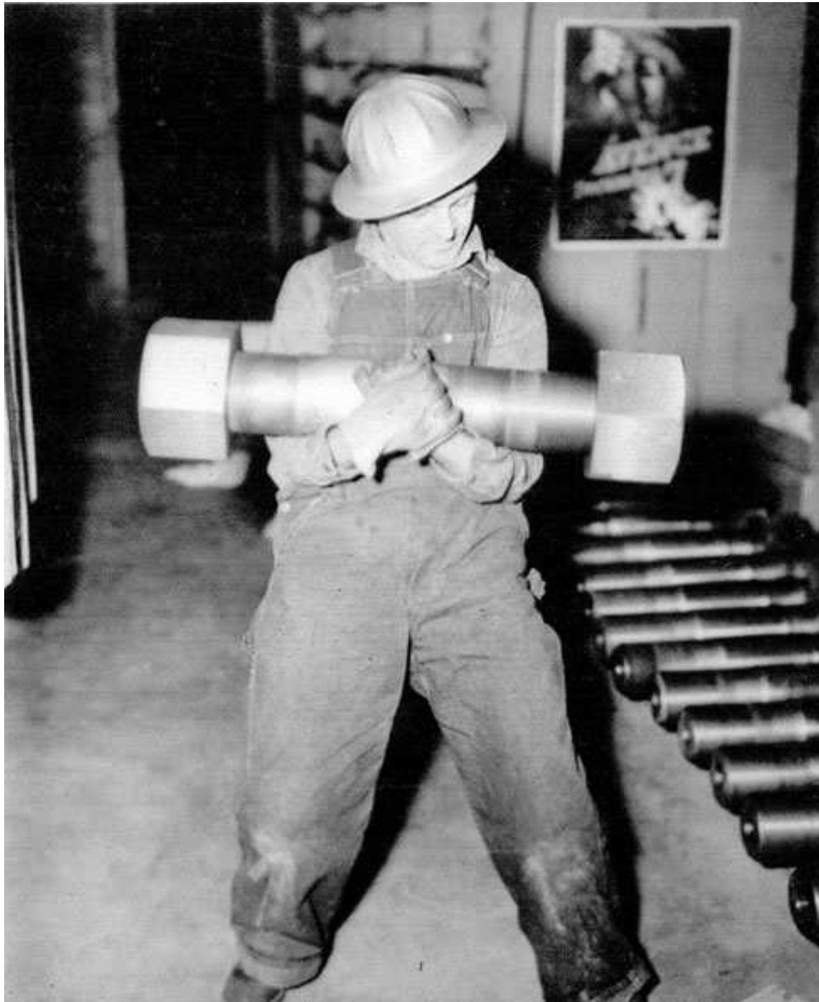
Left: caption: “These 193 lb. bolts and nuts couple the two shafts together on a main unit at Grand Coulee Dam, December 1942”
