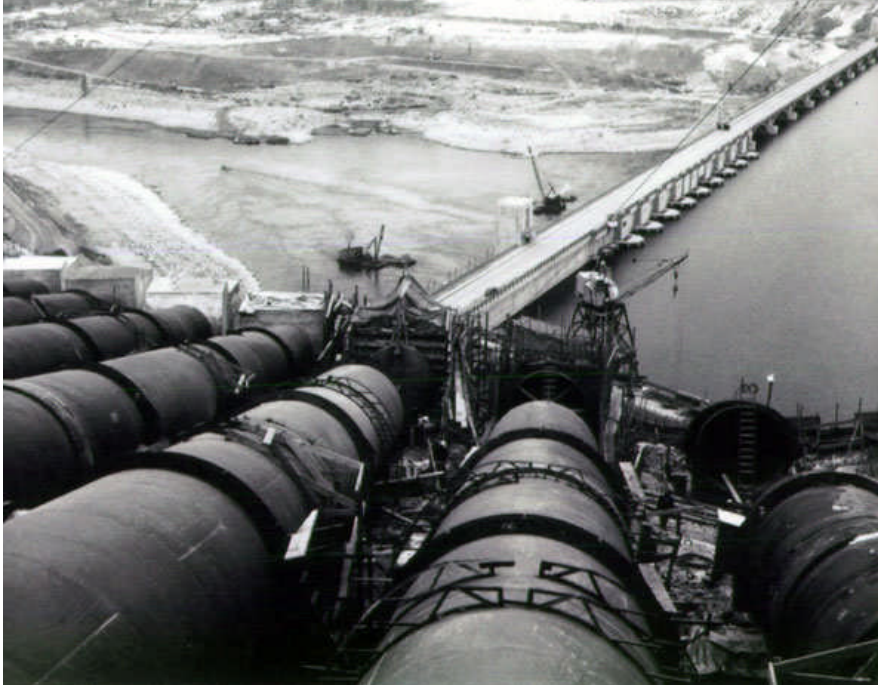
Top Left: caption: “Nine of the twelve discharge tunnels for the pumping plant seen here on the west side of Grand Coulee Dam (August 1938)”
