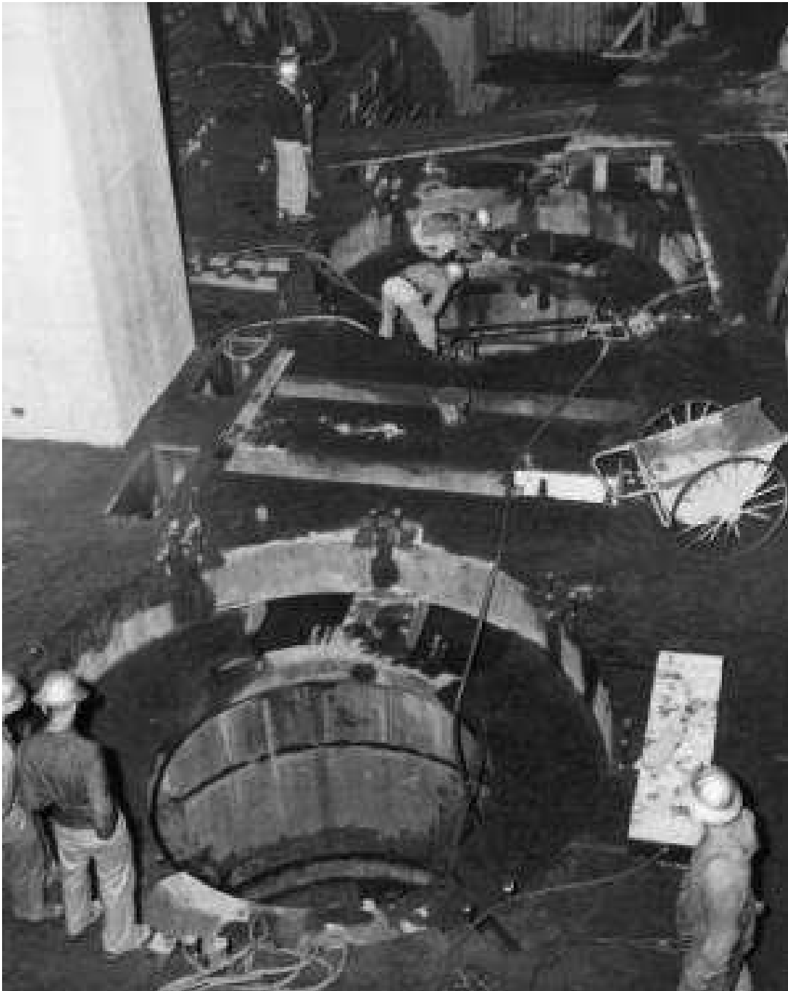
Above: caption: “Scroll case ready for concrete in L-9 turbine pit at the west powerhouse of Grand Coulee Dam (December 1947)”
