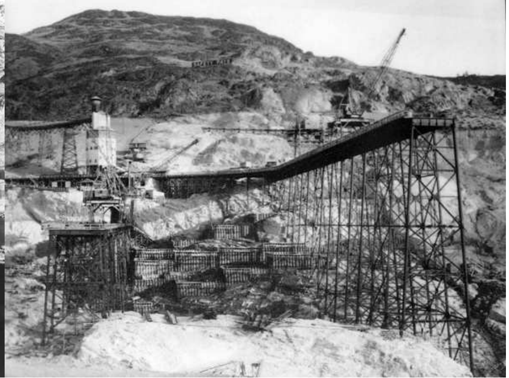
Top Left: caption: “Looking northeast over west side high and low crane trestles, note the cantilever cranes, at Grand Coulee Dam (November 1936)”
