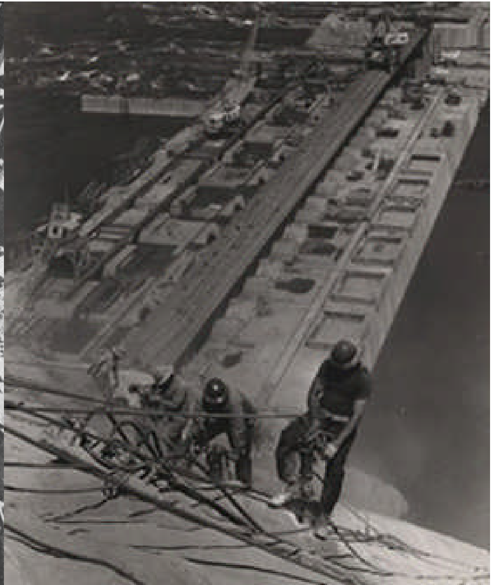
Above: caption: “Jackhammer crews drilling blasting holes at Grand Coulee Dam, 1938”
