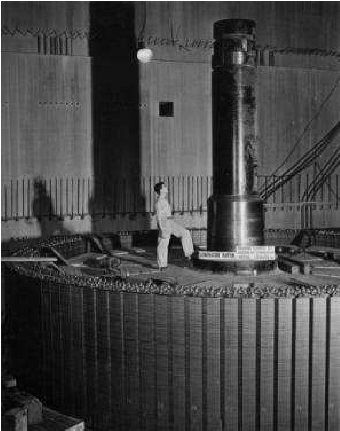
Above: caption: “Lowering the L-7 rotor into place, February 1942”
