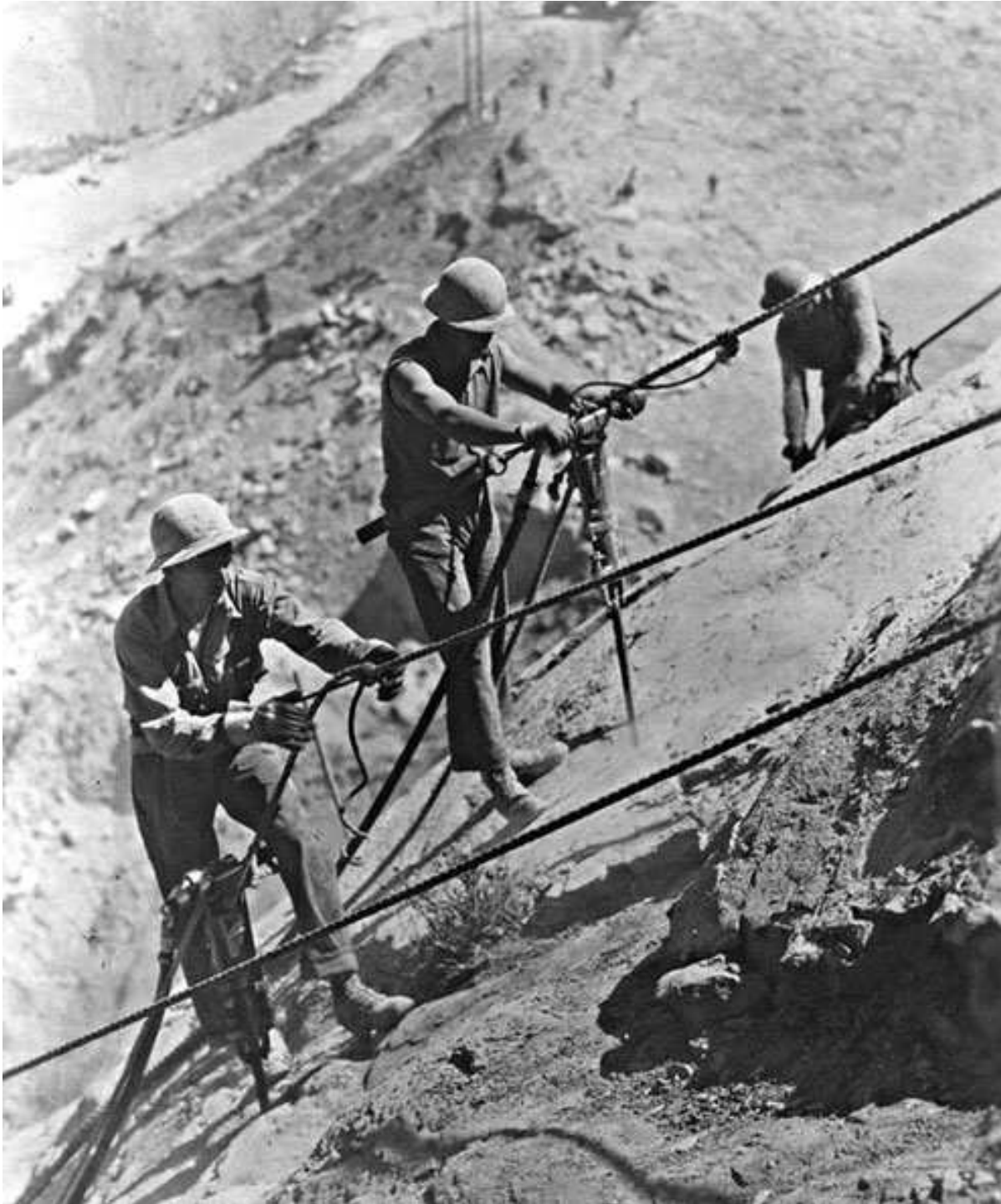
Above: caption: “Drilling blasting holes in rock face for Grand Coulee Dam (ca. 1938)”
