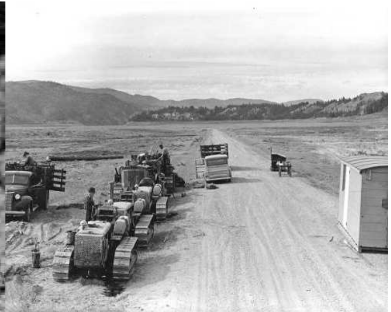
Above: caption: “Caterpillar tractors used by WPA in clearing the Grand Coulee reservoir are shown lined up for service beside the old Highway-22 on the flat midway between the towns of Daisy and Rice, during final clearing operations in the Camp Gifford area. Lake water formed by the Columbia river backing up behind Grand Coulee dam will soon cover this area.”
