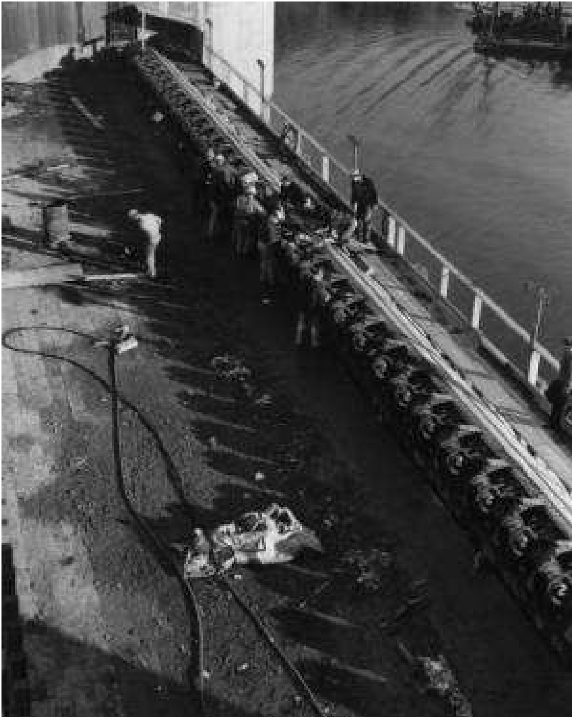
Above & Left: caption: “Men align drum gate hinges, Nov. 1940”
