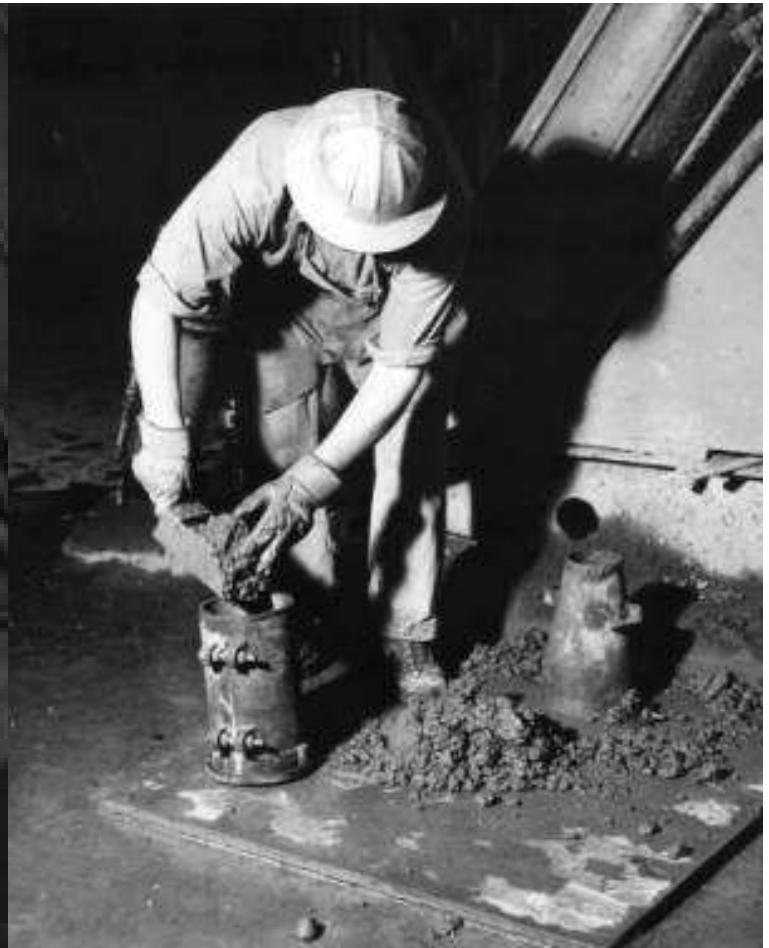
Above & Left: caption: “Gov’t. inspector filling cyl- inder with concrete sample at plant for slump test, June 1940”
