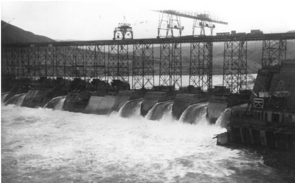
Top Left: caption: “Looking northeast over west side high and low crane trestles, note the cantilever cranes, at Grand Coulee Dam (November 1936)”
