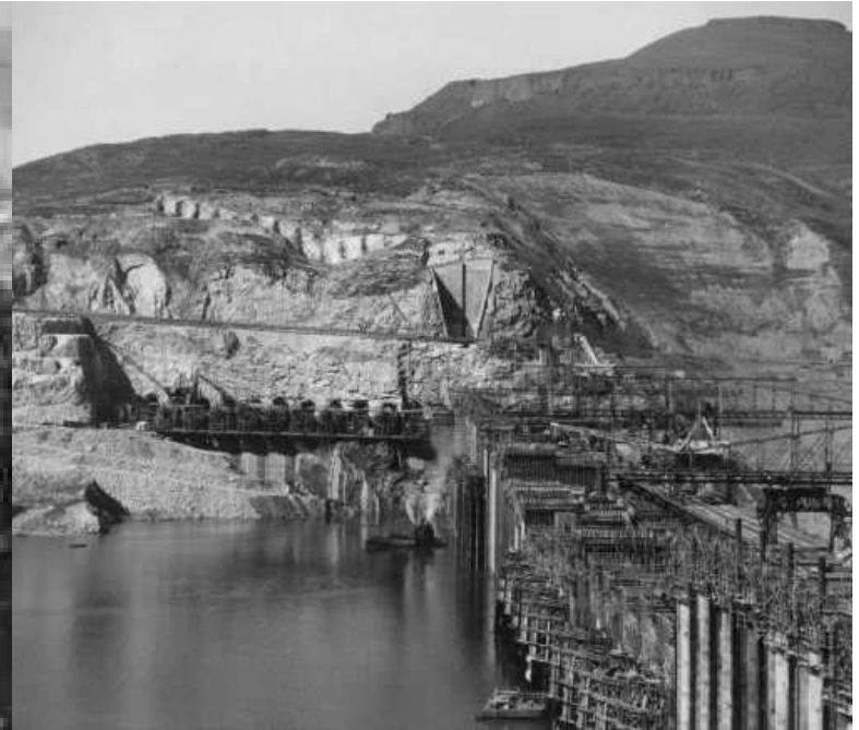
Above: caption: “Coulee Dam irrigation pumping plant and discharge pipes – west crane recess, April 1940”
