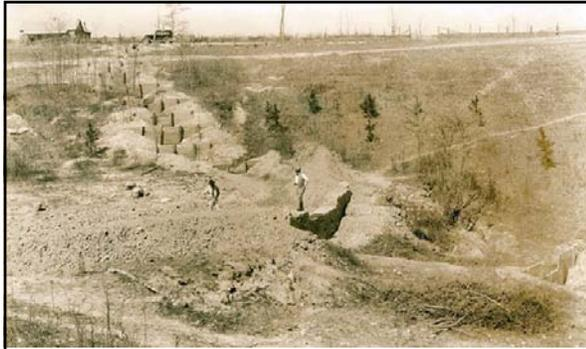
Above: caption: "CCC Tennessee Soil Erosion Project. "Improper disposal of the drainage from the highway caused the erosion in the head of a farm near Demoray. Plank check dams were built in the main gully, with a masonry soil-saving dam constructed at a point where it would catch a considerable amount of silt. The further treatment of this area will be to plant locust and pine." 319
