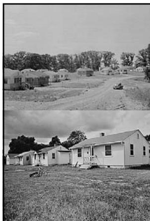
**"...In the field of housing, the TVA offered the war program the results of eight full years of experiment in providing homes for workers. The authority's demountable house, complete with electric, water, sanitary and other installations, is designed for trailer transportation and can be erected in four to six hours..."**
