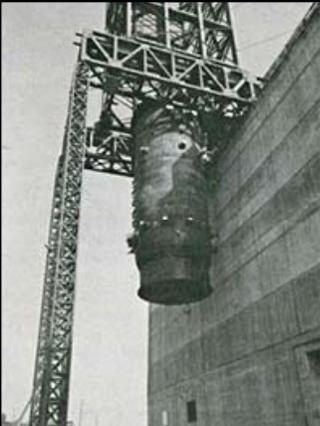
***"...A nuclear reactor is simply an apparatus in which a chain reaction, the splitting of atoms to produce heat, can take place with precision and safety. The heat can be controlled by regulating the nuclear reaction. The reactors for the brown's Ferry plant use water as a means to absorb heat from the nuclear reaction to produce steam. The steam turns the turbine-generators that generate electricity..."***
