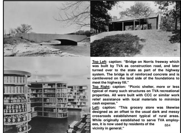
**Top Left:** caption: "Bridge on Norris freeway which was built by TVA as construction road, and later turned over to the state as part of the highway system. The bridge is of reinforced concrete and is cantilevered on the land side of the foundations to meet the highway fill."
