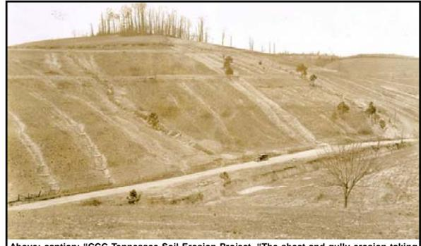
Above: caption: "CCC Tennessee Soil Erosion Project. "The sheet and gully erosion taking place on the Ford farm near Alder Springs Exchange was checked by means of diverting the water into one channel into which plank and masonry check dams were built. The other gullies were plowed in, seeded to grass and small bag dams placed crosswise the gully to prevent any wash taking place prior to the grass becoming established. This area is to be planted to trees as a further means of control." 320
