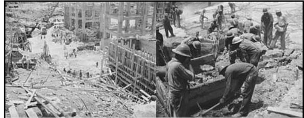
*"...The geologists go to work again on the river-bed, when piles driven in have changed its course so they can work on the bottom where the dam will be. They drill to test the rock and fill in flaws as you'd fill a tooth 'grouting,' they call it; one of the things invented on the job at Norris was a special tool, a sort of feeler, for this purpose. They're so sure of what is under the dams that they draw pictures of it..."*
