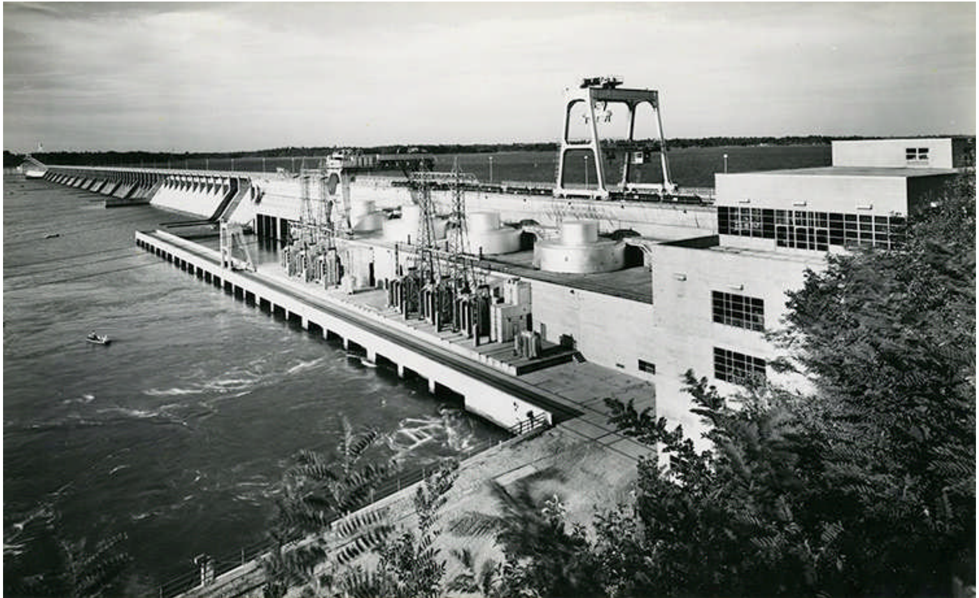
Above: caption: “The Wheeler Dam project was the first main-river dam built by the Tennessee Valley Authority, and one of the few visited by President Roosevelt (February 1934)”
