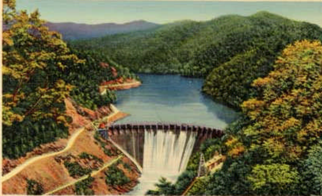
21 Cheoah Dam, Tapoco, North Carolina, near Great Smoky Mountains National Park
