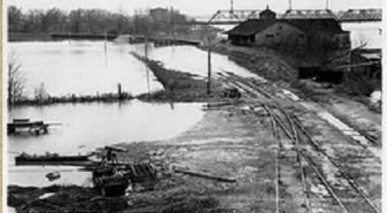
Johnsonville, Tenn., Tennessee River, Gage 33.5', 2-5-37. Portion of railroad track in T.L. Herbert and Sons loading yard was flooded. 13349
