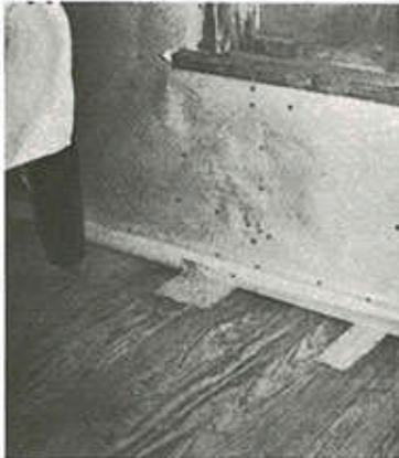
cover wall cracks with heavy paper,
