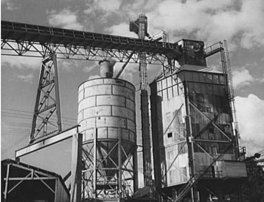
Top L&R: caption: “Aggregate storage pile which provides crushed stone and sand for the building of the new Fort Loudoun Dam, furthest upstream of the TVA’s main Tennessee River projects”
