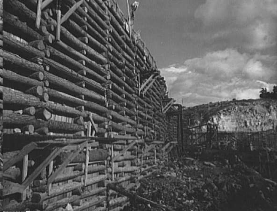
Top Left: caption: “Logs for the construction of a cofferdam at TVA’s new Douglas Dam on the French Broad River”
