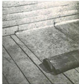
and cover floor cracks with roofing paper.
