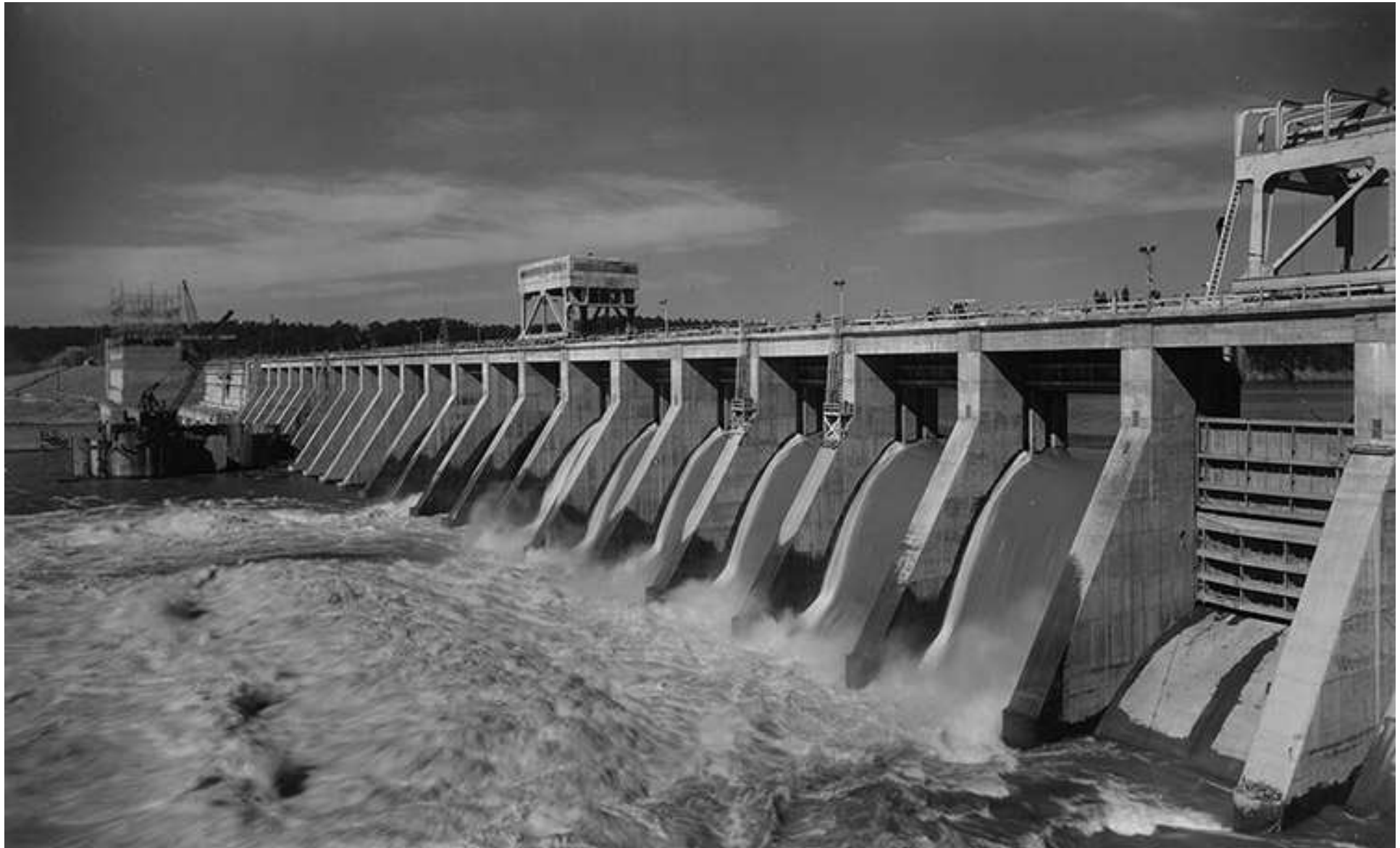
Above: caption: “Pickwick Dam was constructed between 1935 and 1938 and was named for the nearby community at the time. Along with Wilson and Wheeler Dams, Pickwick flooded the Muscle Shoals area which significantly impeded Tennessee River traffic prior to the 1930s (March 1938).”
