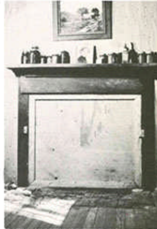
seal fireplaces so mos- quitoes that fly down chimney cannot get in,
