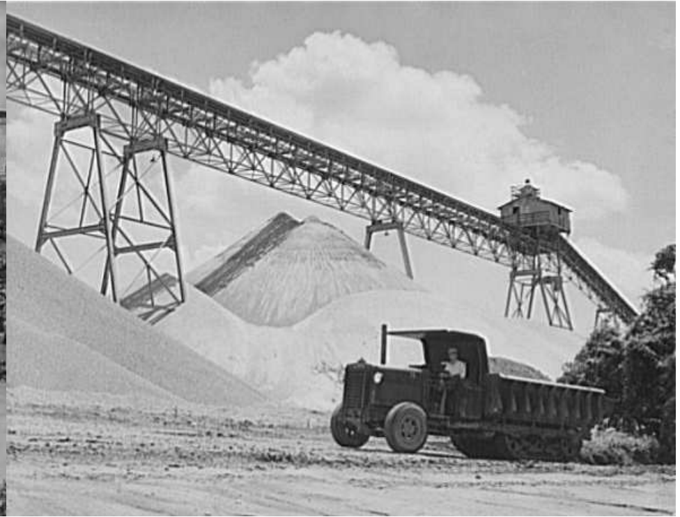
Top L&R: caption: “Aggregate storage pile which provides crushed stone and sand for the building of the new Fort Loudoun Dam, furthest upstream of the TVA’s main Tennessee River projects”
