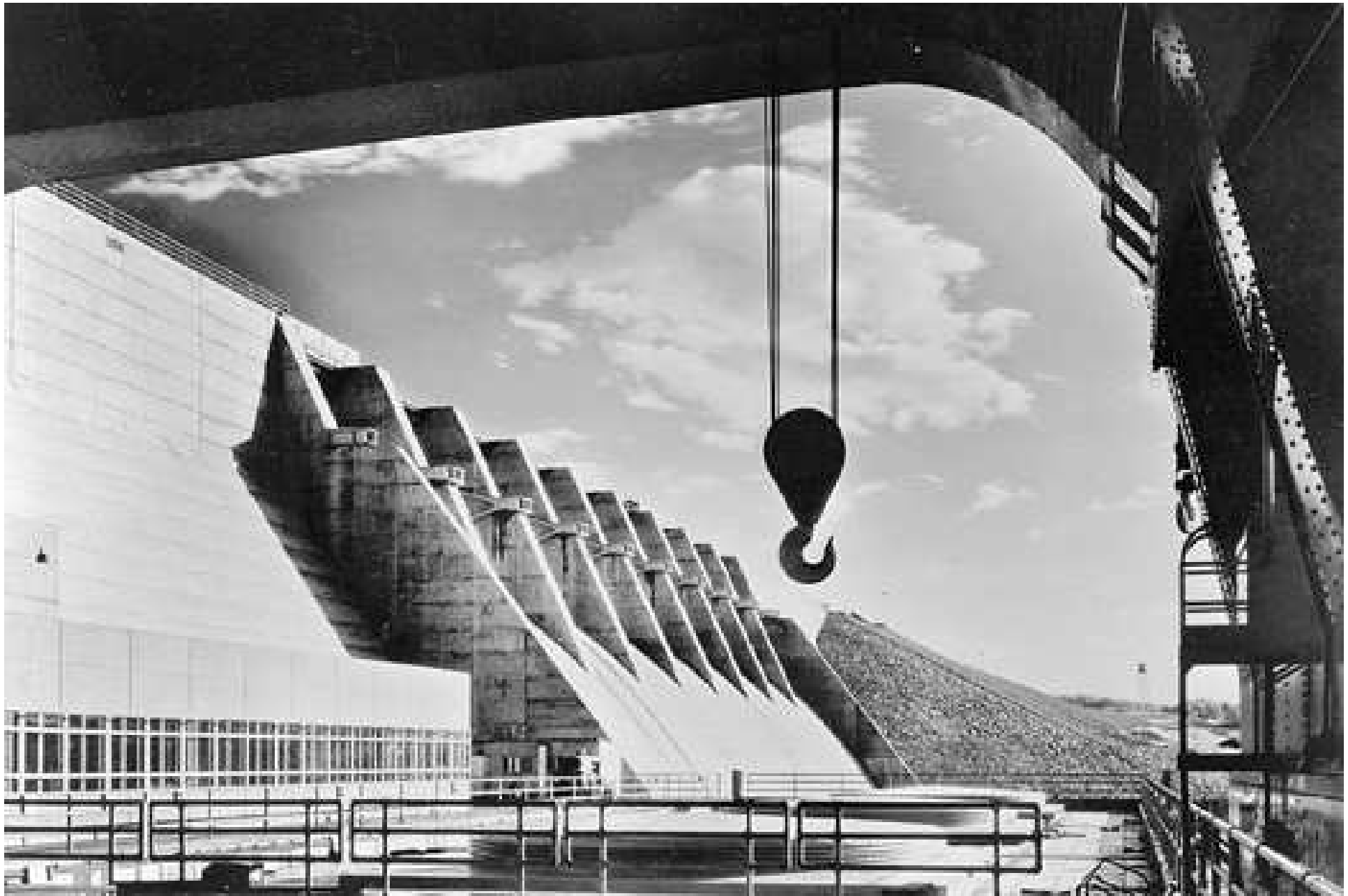
Above: caption: “The TVA built Cherokee Dam on the Holston River in the early 1940s to help meet urgent demands for energy at the outbreak of WWII” 658
