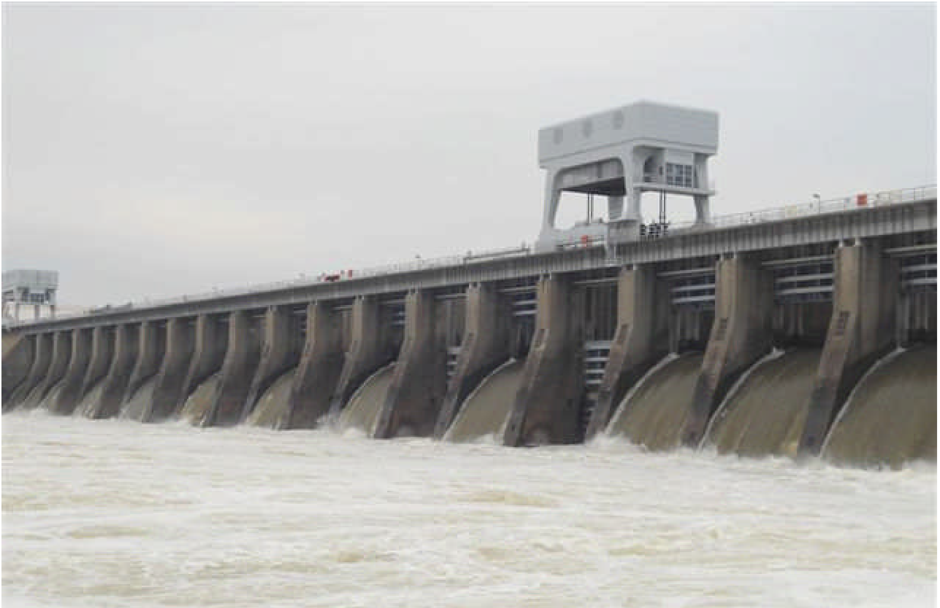
Above: caption: “TVA built the Kentucky Dam in the late 1930s and early 1940s to improve navigation on the lower part of the Tennessee river and reduce flooding on the lower Ohio and Mississippi rivers”
