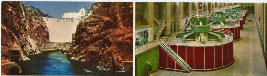
INSIDE DAM—32,500 KVA GENERATORS
