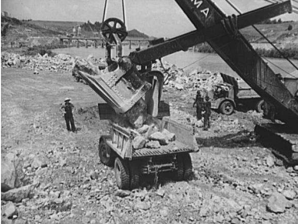
Top Left: caption: “Loading out rock for crushing into aggregate for concrete work at TVA’s new Douglas Dam on the French Broad River”
