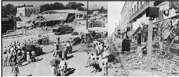
Left: caption: "Main Street, Tehachapi, after the earthquake of July 21, 1952. The two-story concrete (with wood floors and roof) structure in the background is the Catholic Youth Center. Despite the fact that most of Tehachapi's business section was at least partially destroyed, this building suffered little damage."
