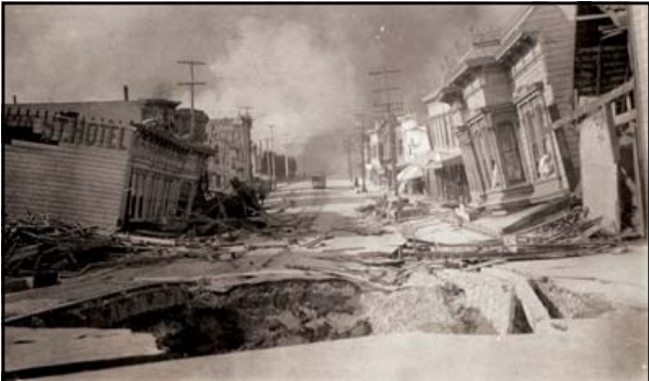
"...Contrary to popular belief, the earth doesn't open up and swallow houses or people. Large fissures are rarely opened up by quakes and these almost invariably remain open. ..." Popular Mechanics, July 1935 335 Above: caption: "Valencia Street after the 1906 San Francisco earthquake"
