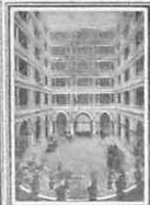
The City Hall, one of the most magnificent structures in the city, was destroyed by the earthquake and fire.
