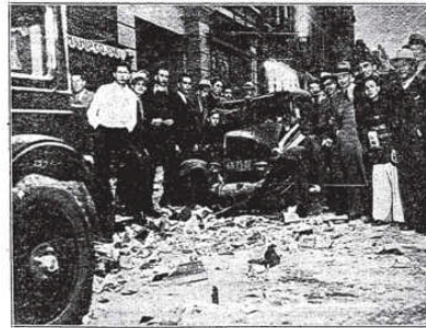
Result of Toppled Cornice in Downtown Los Angeles.
