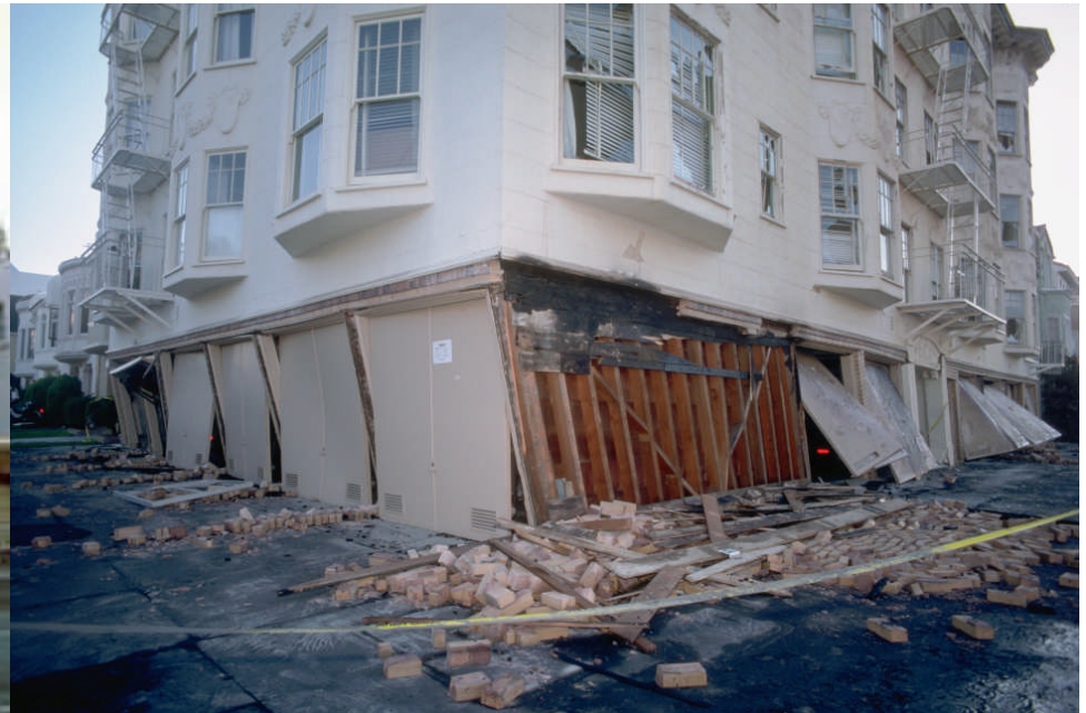
Above & Left: caption: “Many soft-story wood-frame buildings were damaged in the 1994 Northridge earthquake (left) and the 1989 Loma Prieta, California earthquake (top L&R)”
