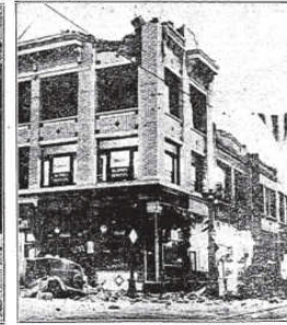
Damage to Building in San Pedro. —Walt Photo.
