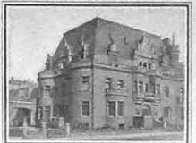
The house which was destroyed by the earthquake and fire, one of the most magnificent structures in the city.
