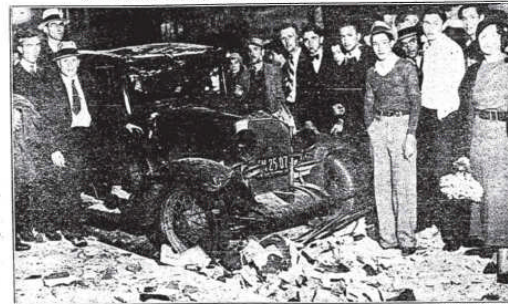
Falling Bricks Wrecked This Car in Downtown Los Angeles. —Walt Photo.
