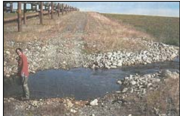
Above: caption: "Plate 5 - Typical low-water crossing with armored banks, widened pool at vehicle ford, and constricted outlet which helps prevent blockage at low flow (Polygon Creek, MP99.0)"
