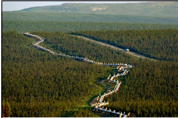
Above: caption: "When the first warm oil was put in the pipeline during start-up in 1977, the above-ground pipe lengthened almost 4-feet per mile. A straight pipeline would not have the flexibility to absorb that much growth." 715
