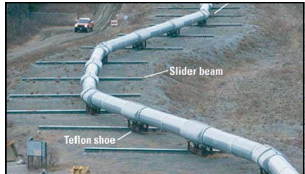
Above: as the elevated pipeline approaches the Denali Fault, it comes off its Vertical Support Members (VSMs), the H-shaped pilings that hold the pipe above ground in the permafrost zone. The pipe is placed in a steel shoe, which sits on top of a low-to-the-ground concrete beam. The bottom of the pipe shoe is covered in a slippery, Teflon-coated plate, allowing it to slide across the beam. At the Denali Fault, the pipe can slide up to 20-feet horizontally and 5-feet vertically. 720
