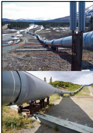
"...At the Denali Fault, support beams allow sideways slippage of 20 feet and a vertical drop of five. 'Any quakes that would disturb things more than that,' says Dennis Knottingham of R&M Consultants, an Anchorage bridge-design firm, 'are projected to happen only once every two centuries.' Adds Mr. Champion: 'You just couldn't develop a better system for handling earthquakes'..." Popular Science, April 1977 Left T&B: caption: "Trans-Alaska oil pipeline at the Denali Fault crossing" 719
