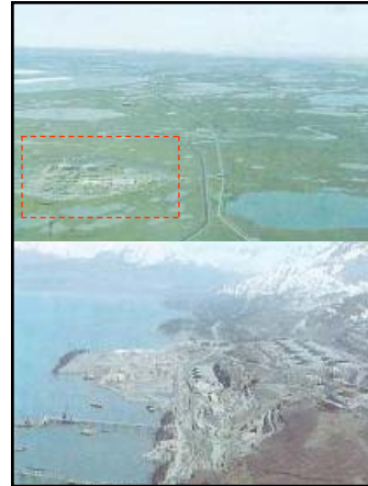
Top: caption: "Plate 27. Pump Station 1 built in wet-meadow tundra (HQ) about four miles south of Prudhoe Bay in A.S. 138, Section 6. View is northwest. A lake of approximately 140 surface acres in size was drained so that this pump station could be constructed. July, 1977."
