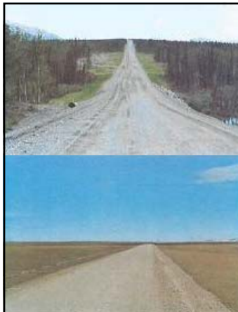
Top: caption: "Plate 15. A portion of the Haul Road constructed through spruce-deciduous woodland (HMQ) in A.S. 97, Section 4. View is north. Note new growth on the cut and fill slopes from revegetation with grasses. June, 1977."
