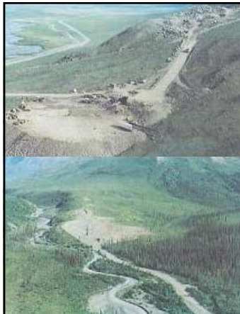
Top: caption: "Plate 31. M.S. 112-3.1 and a disposal area built in tussock tundra (MQ) and alpine tundra (LMQ) on the north side of the Brooks Range, A.S. 112, Section 5. View is north. An access road leads to site. Work pad lies between the Atigun River and the Haul Road in photo background. June, 1976." Bottom: caption: "Plate 32. M.S. 108-2 located primarily in subalpine (MQ) habitat, A.S. 108, Section 5. An access road from the Haul Road was constructed through shrub thicket (HMQ) and spruce woodland (LMQ). View is west. June, 1976." 579
