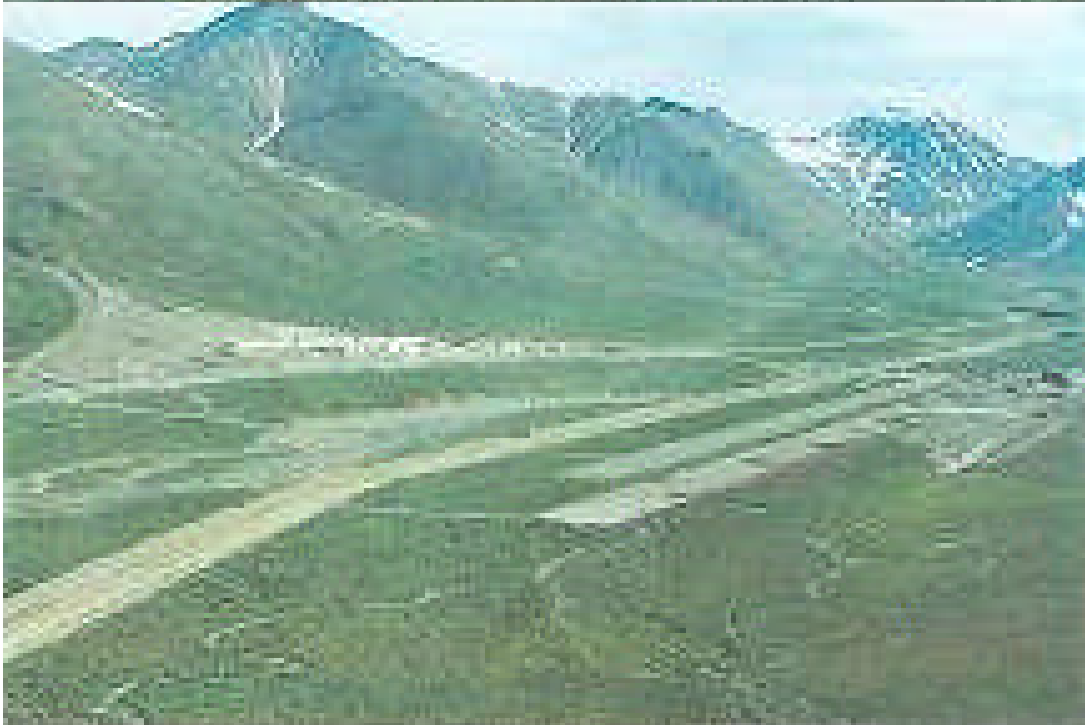
Bottom: caption: “Plate 26. Chandalar Camp built in subalpine (MQ) and riparian willow (HMQ) habitats, A.S. 109, Section 5. View is north toward the Continental Divide in the Brooks Range. Access roads from the Haul Road can be seen coming down to the work pad in the North Fork of the Chandalar River. The camp airstrip is located between the work pad and M.S. 109-3 (right side of photo). June, 1976.”
