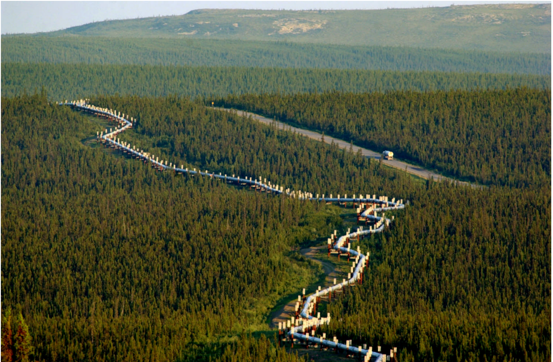
Above: caption: “When the first warm oil was put in the pipeline during start-up in 1977, the above-ground pipe lengthened almost 4-feet per mile. A straight pipeline would not have the flexibility to absorb that much growth.” 715
