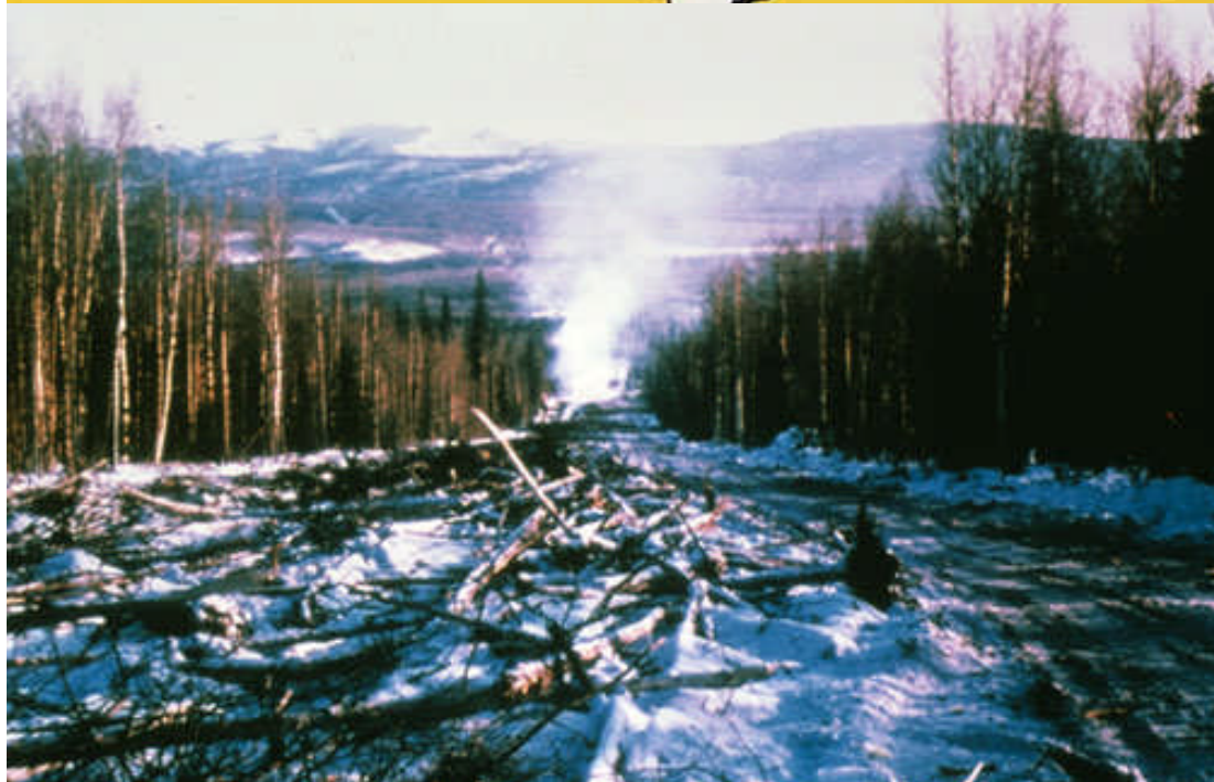
Bottom : caption: "Winter Haul Road under construction, 1969"
