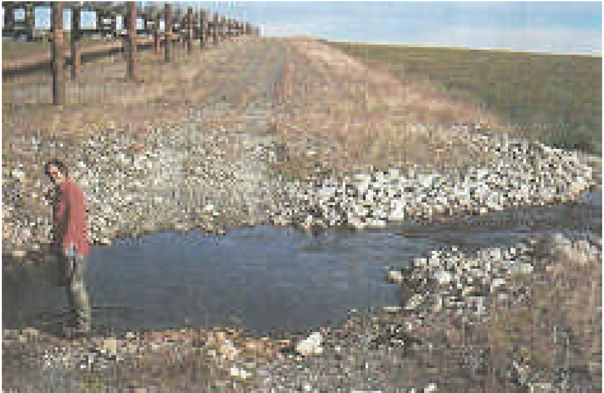
Above: caption: "Plate 5 - Typical low-water crossing with armored banks, widened pool at vehicle ford, and constricted outlet which helps prevent blockage at low flow (Polygon Creek, MP99.0)"
