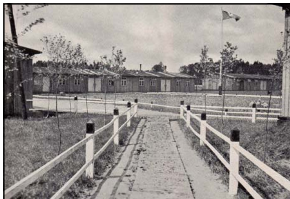
Fig. 2. View into inner court of Labor Camp near an autobahn working place. Eastern Prussia
