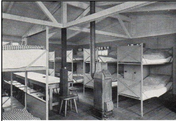
www.PDHonline.org www.PDHcenter.com 577 Fig. 3. Sleeping Room with Heating
