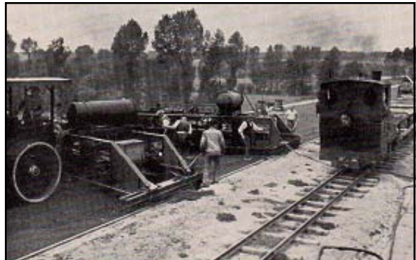
Fig. 12. Consolidating of bituminous surfaces by roller and vibration finisher
