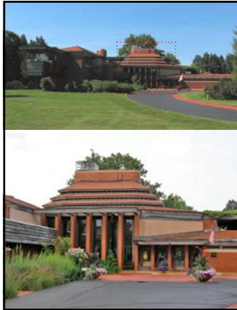
Left T&B: at the center of this front view of the house is the Central Core (highlighted) with the bedroom wing to the left and guest room/garage wing on the right. Atop of the central core is one of the most distinctive features of the house; an observation cupola FLW added for the children to be able to watch their father's plane approach when he returned from trips. The brick was the same used in the Administration Building.
