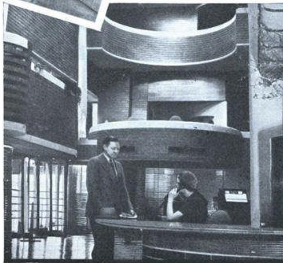
Center, glass-enclosed bridge linking two buildings. Above, glimpse of tapering "golf tee" columns which support roof. Circular stairways between floors save space. Reception hall is seen below
