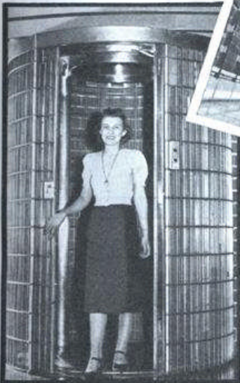
Above, the circular "bird-cage" elevator. Radiant floors heat the building, steam pipes being laid under the four-inch concrete slab. Without a conventional front door, entrance is through a roofed-over auto driveway. Near by is a "carport" for parking, and on its roof a theater and a squash court
