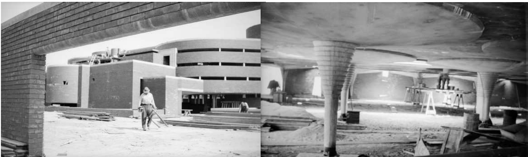
Below Right: caption: “Tapered columns in the Johnson Wax Building during construction. Workmen are working on scaffolding built around one of the columns.”
