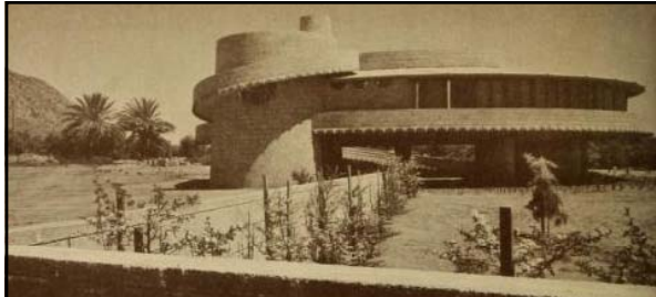
Above: caption: "1952. Patio house in the Southwest, Phoenix, Arizona – for son David Wright. David himself supervised the construction using concrete block made by the Besser machine. It is a good type of house for that region and affords many advantages not possible to a house on the ground. It is a citrus orchard district and the orange trees make the lawn for the house. The slowly rising ramp reveals the surrounding mountains and gives security to the occupants. The house is completely in masonry with mahogany ceiling and sash frames and doors. A small roof garden reached by a minor ramp surmounts the whole. The house is roofed with copper green enameled sheet iron in appropriate pattern." Excerpt from catalog of an exhibition held October 22nd - December 13th 1953 at the Solomon R. Guggenheim Museum, NYC entitled: "Sixty Years of Living Architecture: The Work of Frank Lloyd Wright." 315
