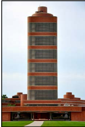
"...Where the Administration Building seeks to convey an impression of extreme horizontality, what came to be called the Research Tower is obviously intended to provide a strong vertical contrast; sturdily square in plan but with rounded corners, it rises with the dignity of a miniature skyscraper. It is clad in alternating bands of brick and obscure glass tubing, through the glass one is able to detect that the building consists of a central mast, from seven square shelf-like floors project, each of them of sufficient height to contain a circular mezzanine level. The floors extend to the cladding, while the mezzanines, which are in effect free-standing, permit, by Wright's reckoning, an ease of oral communication between workers on the two levels. Fitted with the mast are a circular elevator, fire stairs, and utilities..." RE: excerpt from Many Masks: A Life of Frank Lloyd Wright 295
