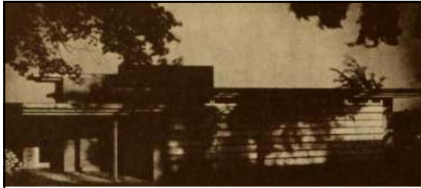
Above: caption: "1934. The first Jacobs house – wood walls and ceilings. Although used in the Imperial Hotel, Tokyo, 1914, and subsequently planned for the Nakoma Clubhouse, 1927, and the Johnson Administration building, 1935, gravity-heat was first a finished product in this house. Therefore this was the first floor-heated house in the United States." Excerpt from catalog of an exhibition held October 22nd - December 13th 1953 at the Solomon R. Guggenheim Museum, New York City entitled: "Sixty Years of Living Architecture: The Work of Frank Lloyd Wright." 223
