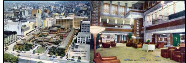
"...The fact is that, despite their flaunting of all acceptable standards of architectural soundness, Wright's buildings have shown both astonishing practicality and remarkable durability. The Imperial Hotel in Tokyo, built like a vast float riding on a jellylike foundation of mud, has, in fact, survived some of Japan's worst earthquakes and has sustained its only injuries recently under the pounding of American bombs..." LIFE magazine, August 12th 1946 Above L&R: postcard featuring the Imperial Hotel (ca. 1950s) 140
