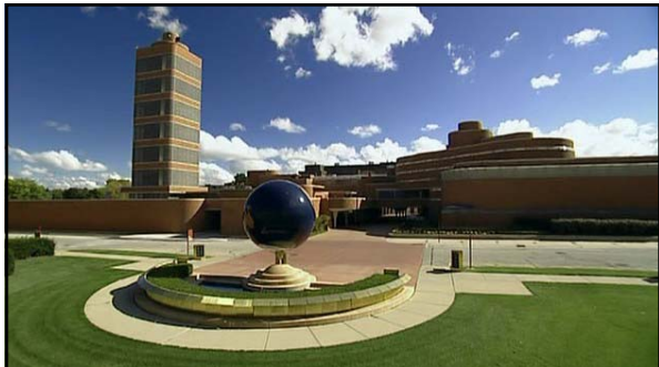
"Whenever Frank Lloyd Wright designs a building, you can be sure it'll be different. Usually it is also good looking and functional. This, one of the newest, is no exception..." Popular Mechanics, January 1950 RE: SC Johnson & Company Research Tower 297
