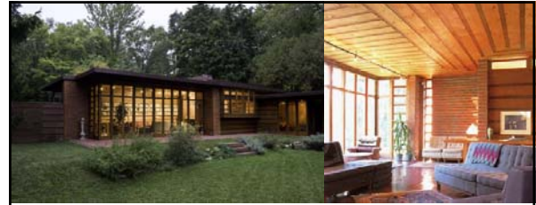
"...He called his modest house 'Usonian,' after the United States. It was a single story built on a monolithic concrete slab and joined to a carport and not a garage. Wright believed that it could be replicated all across the country. His main desire, which no contemporary architects pay any attention to whatever, is shelter for ordinary people...he got it down at one point in 1940 to $5,000 per house for a family with children and a kitchen and gardens...and openness and a real milieu in which it was a highly civilized way to live. He thought about it all the time; he took commissions from the poor as well as from the rich...We're not like that anymore and this was very important in any appraisal of what his work represents because he hasn't had the following that he should have had in respect to shelter..." Brendan Gill, Writer/Author 224 Above L&R: exterior/interior views of FLW's Usonian (Jacobs I) house
