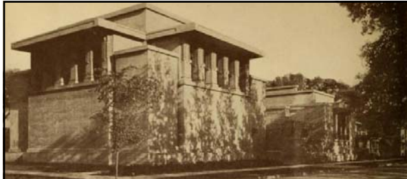
Above: caption: "1906-07. Unity Temple, Oak Park, Illinois. So far as I know the first concrete monolith to come from the forms as architecture completely finished. The work was cast in wooden forms or boxes – and the forms bear the impress of that technique. The plan first began the destruction of the box, and the emphasis of interior space as the reality of the building subsequently carried on. The entrance is between the temple and the secular rooms. Here electric lighting took visible form in wiring and became a decorative feature of the structure." Excerpt from catalog of an exhibition held October 22 nd - December 13 th 1953 at the Solomon R. Guggenheim Museum, NYC entitled: "Sixty Years of Living Architecture: The Work of Frank Lloyd Wright." 85
