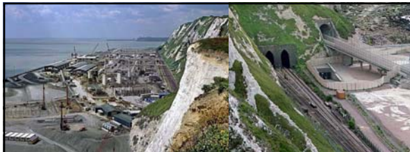
Left: caption: "The Channel Tunnel construction site in June 1991. The site required for the Channel Tunnel construction was considerably more than the former colliery site. This required land to be reclaimed from the sea. To do this, steel sheets were driven into the sea bed to make a coffer dam; this was subsequently filled with concrete. The enclosed area was then pumped out and filled with sand."
