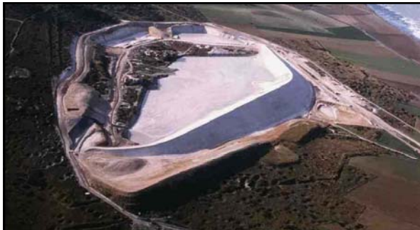
"...On the French end, the spoil was mixed with water, then this slurry was pumped out and dumped behind a 132-foot-tall dike. This mountainous, soggy heap should finally solidify in 1995; it will then be landscaped as a park..."
