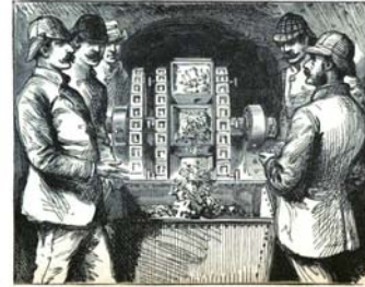
EXAMINING THE BORING MACHINE.
