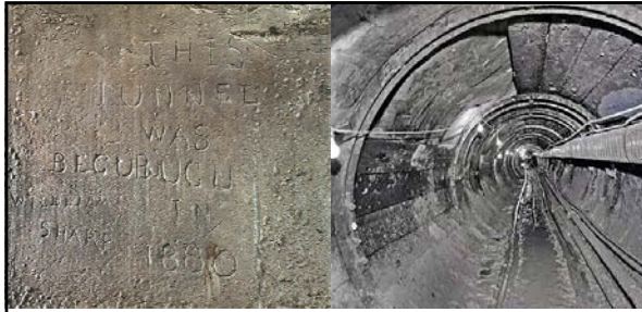
In 1880, under the direction of Sir Edward Watkin, Chairman of the South Eastern Railway, a new shaft (No. 1) was sunk at Abbot's Cliff (between Dover and Folkestone) with a horizontal gallery being driven along the cliff (10-feet above the high-water mark). This seven-foot diameter pilot tunnel was eventually to be enlarged to accommodate standard gauge railway tracks, with a connection to the South Eastern Railway. Left: inscription by miner William Sharp, recording the start of tunneling Right: the 7-foot diameter pilot tunnel (dewatered in 1988)
