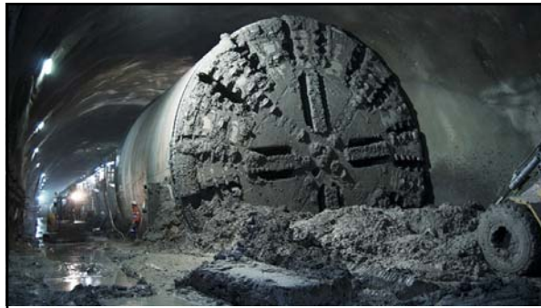
"...When the grinding face is pulled away from the tunnel end so that worn teeth can be replaced, if you carefully climb forward you can glimpse the chalk marl, the color of dirty tennis shoes. It looks awfully solid. It's grooved like a target, dug out by 236 tungsten-carbide gouging bits on the grinding plate. They form a star pattern on the machine's face - like a colossal sand dollar..." Popular Science, June 1990 1261
