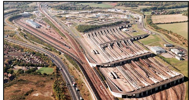
"...When Folkestone citizens drive by the new terminal site they remember what it used to be: 'Beautiful country fields with sheep,' recalls Eric Pratt, a phone company trouble-shooter. 'Lovely little houses by a picturesque stream. Now there's not even a dip.' The land was leveled with 6.6 million cubic yards of sand dragged from the channel then slurried up through culverts..." Popular Science, June 1990
