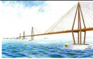
The great vertical supports and cable stays of EURO ROUTE's bridge sections.
