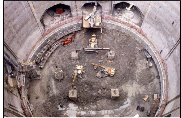
Above: caption: "Channel Tunnel construction – Sangatte access shaft from above, July 1987"
