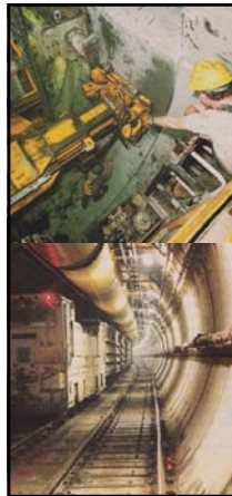
"...As the waste rumbles out, precast concrete tunnel sections ride in. They're hard (12,000 psi, four times the compression strength of standard bridge concrete) and smooth. Run your finger along their surface and they feel like marble. They vary in thickness from 6.5 to 20 inches and weigh up to nine tons each. 'It depends on the maximum possible overburden pressure,' explains Stacey. 'We say, how far is it to the surface of the water? And then determine the strength as though the overburden were mud.' The crescent cement slices are set into place by five men directing hydraulic lifters with hand-held switch boxes. The last section is a shaped keystone, shoved snugly into place by one of the rams. The tunnel diameter shrinks to 24 feet..." Popular Science, June 1990
