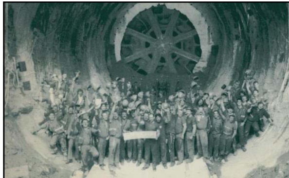
Above: caption: "November 20, 1990: Folkestone. Another milestone was reached today in the building of the Channel Tunnel when the final underground section between the Kent coast and the terminal site broke through. The workers are pictured celebrating their arrival in Folkestone."
