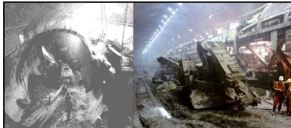
The cavern was formed in stages with side headings, crown, bench and invert sections using sprayed concrete temporary and permanent linings. At the time of excavation, this was the largest undersea cavern ever built, representing a major technological tour-de-force . Left: caption: "Excavating the French Crossover to reveal the already-built tunnel" Right: caption: "Running tunnel TBM in Crossover" 1593
