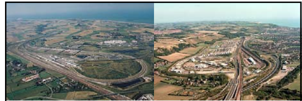
Left: caption: "Covering an area of 650-hectare and 23-km long perimeter, the Coquelles terminal, near Calais, is one of the largest land-travel complexes in Europe (the equivalent in size to an international airport). As a result of the marshy nature of the soil, the whole area had to be covered with a 50-cm thick layer of sand before construction could begin in order to ensure a good base for the foundations."
