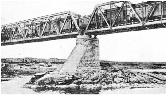
"...For the reinforcement of the piers they introduced triangular buttresses pointing upstream, on which the ice broke and divided, instead of piling up and causing serious damage to the structure as a whole..." Wonders of World Engineering, June 8-15, 1937 Caption: "ONE OF THE MANY BRIDGES which are a feature of the Trans-Siberian railway. Note the reinforced pier which breaks-up ice flows in the river."
