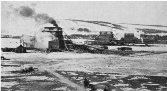
“...Where masonry piers were set up during the winter months, the builders had to protect the unset concrete and mortar from the intense cold by huge wooden sheaths as they progressed. Sometimes they even kept the sheathing artificially warmed...” Wonders of World Engineering, June 8-15, 1937 Caption: “Construction of the Yenisei bridge in winter”
