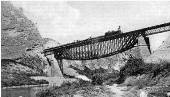
The Siberian Railway is, like all Russian roads, of a five-foot gage. It is constructed after the manner of American Western railways, single-tracked, gravel-ballasted, where ballasted at all, with Howe truss bridges over the smaller waterways, and steel bridges across the large rivers. Caption: "Inverted Bowstring truss bridge across the River Zouriazan"
