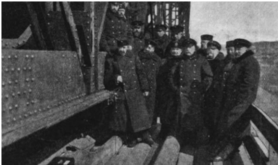
The manner of testing these massive structures is to let four or more locomotives with a loaded train of cars stand on a bridge for several hours, and then to run them back and forth a number of times at a constantly increasing rate-of-speed, till the maximum is reached. Caption: "Bridge bend tested by the Frenkel apparatus"
