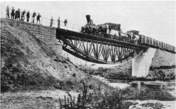
Caption: "CONSTRUCTION TRAIN, drawn by two wood-burning locomotives, with a trainload of materials for the laying of the Trans-Siberian Railway. The train is crossing over one of the early types of bridge used for spanning smaller waterways. In the Mid-Siberian section of line alone 574 bridges had to be built."
