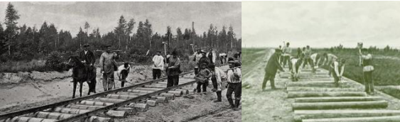
We think, however, that it would have been a wiser policy if the engineers had adopted a better class of track tie. As will be seen from our engraving, many of the tie consist merely of soft-wood trees cut to length and split in two. These are laid with the flat face down and a notch is adzed in each to receive the rails. The weak features of this type of tie are that it presents but small bearing surface for the base of the rail, which quickly cuts down into the tie that is hewed on opposite faces. In one of our illustrations showing the laying of the track, the latter form of tie is used, in another the half-round split tie, and the difference in stability and in bearing surface will be readily appreciated by comparing these two pictures. Left: caption: "Track-laying on the Trans-Siberian Railway; note the cheap, half-round ties" Right: caption: "Grooving the ties for rails"
