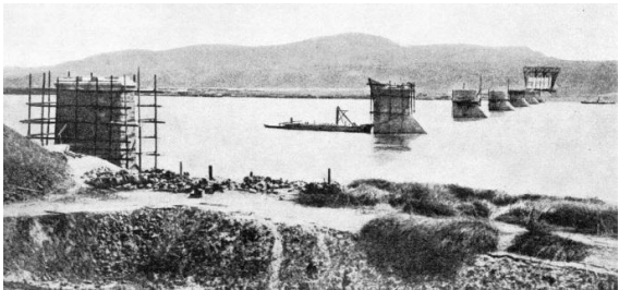
Caption: “BRIDGING THE RIVER YENISEI was one of the biggest tasks in the building of the second subsection of the Mid-Siberian line. Professor L.D. Proskouriakov was responsible for the bridge, which has six spans, each 474-feet-long, of steel girders. The bridge is at Krasnoyarsk, where the Yenisei is normally 2,800-feet-wide. Lack of materials delayed the work for some time, and when masonry piers were set up in winter they had to be protected from the cold by wooden sheaths until the concrete and mortar had set.”
