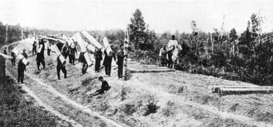
One advantage which this line has over some of our pioneer Western roads, is that the Russians have made very free use of embankments, preferring these to the more hastily-built and less permanent pile trestles, which form such a conspicuous feature of our own Western roads. The earth or rock embankment, once made, requires very little subsequent care, and consequently the great amount of time spent in maintaining ordinary trestle construction will be saved on the Trans-Siberian road. Caption: "Workers carrying timber sleepers to be laid atop earthen embankment in a section of the Trans-Siberian Railway traversing dense rolling woods known as 'taiga'"
