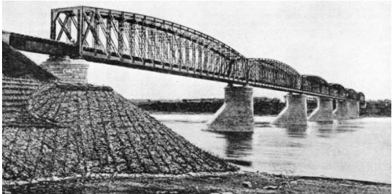
Caption: "SIX STEEL SPANS carry the Trans-Siberian Railway across the River Tom, 103½ miles along the route from Obi. The river here is 1,680-foot-wide, and the six spans of 280-foot rest on masonry piers. The piers are reinforced by triangular buttresses pointing upstream, to break up ice that floats downstream in winter."
