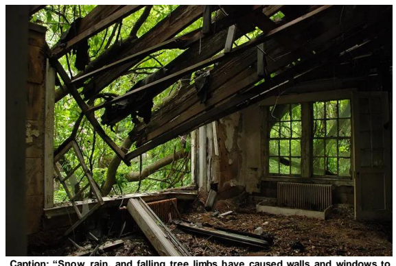
Caption: "Snow, rain, and falling tree limbs have caused walls and windows to cave in. Vines and soil have entered the premises, blurring the boundary between interior and exterior, nature and fabrication."
