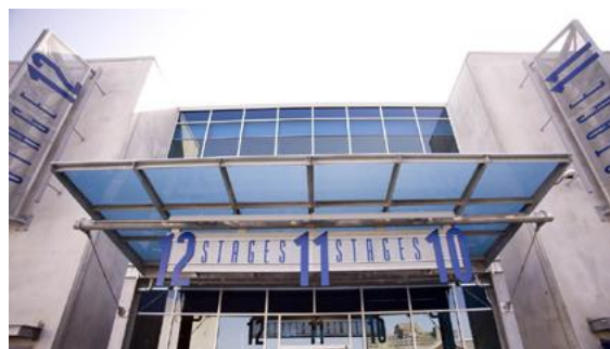
“...The five new stages at Steiner support heavy electrical loads, are soundproof and column-free, and possess massive silent heating, ventilating and air-conditioning units. The building also features various support spaces, offices, dressing rooms, hair and makeup rooms, and wardrobe rooms...”
