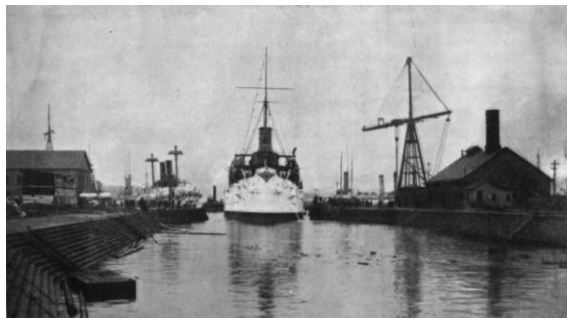
The illustrations which accompany this article will give a clear impression of the construction of these dry docks and the manner in which a warship is carried upon the keel blocks and shored up by struts which rest upon the altars and are wedged snugly against the hull. One of the views shows the cruiser Columbia entering dock No. 2, the caisson gate having been floated away from the entrance, as will be explained later. 487 Caption: "The Cruiser Columbia entering Dry Dock No. 2 at the Brooklyn Navy Yard"
