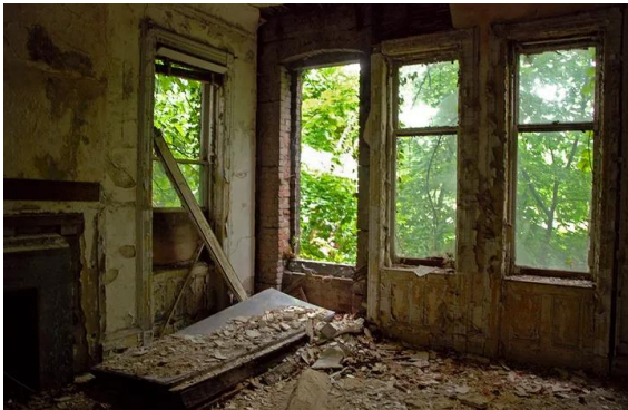
Caption: "'Even where the glass is still intact, rain and snow mysteriously, inexorably work their way under sills,' writes Weisman. 'As the wood continues to rot, trusses start to collapse against each other.'" 1533
