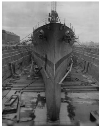
"...When the Department made a new contract for Dock No. 4 with the Williams Construction Company, it enlarged the plans of the old basin. The dock, when completed, will be 601-feet-long. At the entrance it will have a width of 106-feet and in the body of the dock it will measure 110-feet from side-to-side. This will give ample room for the admission of the 25,000-ton 'Wyoming.' The greatest width of this vessel is 95-feet..." The Brooklyn Daily Eagle, July 21, 1909 Caption: "USS Wyoming in Dry Dock No. 4, New York Navy Yard. November 18, 1912." 674
