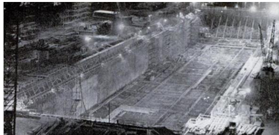
290 Caption: “Its underwater construction completed, the graving dock above has been pumped dry for the laying of a smooth inner surface of concrete. A gate seat is built in the cofferdam in the background.”
