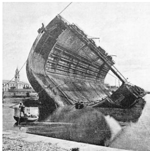
Caption: “THE FIRST BERMUDA DOCK was a hollow-walled iron dock built in 1868. Twenty-four compartments in the walls were pumped dry by eight steam-driven pumps to give the dock a lift of 3,000 tons. To tilt the dock for cleaning purposes, one wall was pumped free of water and the other wall was kept filled. This practice had to be abandoned because there was grave danger of the dock’s capsizing.”
