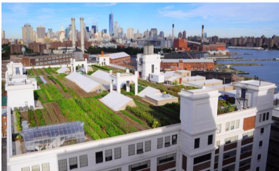
Caption: “Located atop Building No. 3 at the historic Brooklyn Navy Yard, is a massive 65,000 sq. ft. roof towering twelve stories over the East River. Installed in 2012, the farm is covered in 10-12-inches of Rooftite Intensive Ag blend.”
