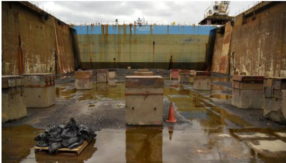
“...A set of blocks waiting for the next customer, as sand blasting debris are cleared away. ‘It’s been very busy, which is good. The busier we are, the more efficient we are,’ says Sanborn. ‘We go through peaks and valleys. I’ve been in this industry for a long time, and we are sort of waiting for it to drop out again. We hope it doesn’t.’” ny.curbed.com, May 3, 2018
