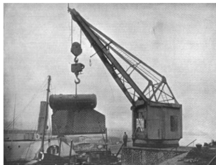
We illustrated a few weeks ago a large crane designed for this purpose, and erected at a German shipbuilding establishment. That crane was of the fixed type, being located at the edge of one of the docks, and, of course, if any ship is to avail itself of its services, it must be warped into proper position alongside the crane.
