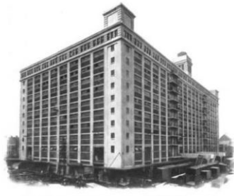
REAR VIEW OF STOREHOUSE, WITH CONCRETE LOADING PLATFORMS AND CONCRETE BRIDGES OVER TRACKS
