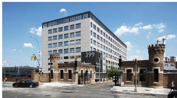
Last December, YIMBY revealed the renderings for 399 Sands Street in the Brooklyn Navy Yard Industrial Park. Now, the official groundbreaking for the nine-story office building has occurred. newyorkyimby.com , June 14, 2018 RE: introduction to an article entitled: "Groundbreaking Ceremony for Steiner's 399 Sands Street, Brooklyn Navy Yard"
