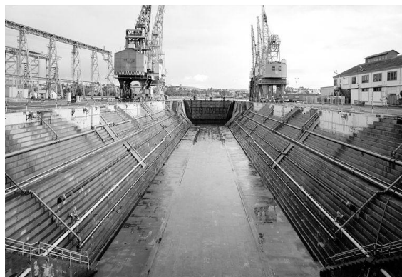
Caption: "Mare Island Naval Shipyard, Dry Dock No. 1, California Avenue, east side near Ninth Street, Vallejo, Solano County, CA" 384
