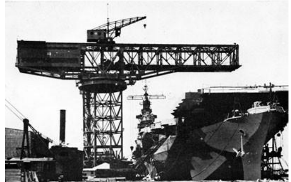
This crane, like its counterpart at Norfolk, was of the turntable type (rather than a pintle crane). Caption: "Hammerhead Crane, Norfolk Navy Yard. This crane was built to provide a 350-ton lifting capacity at a 115-foot radius" 1196
