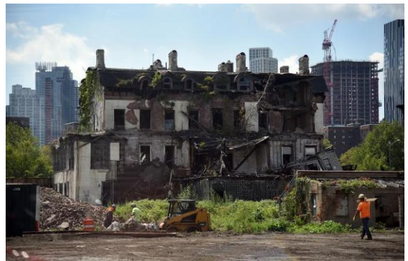
Caption: “Demolition crews preparing the residences at Buildings E, F, and G for destruction. Buildings H and C will also soon be torn down, leaving Building B as the only residence to be preserved”
