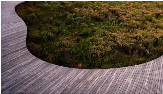
"...Because of the sensitive condition of the site, all structures are designed and engineered with minimal impact upon the landscape. A series of steps and an accessible ramp lead up to the gateway and the level of a raised, wooden walkway..."
