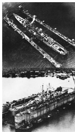
Upper Left: caption: "Cruiser in an ABSD. Showing the ship secured in position so that it will be supported on the prepared blocking as the dock is dewatered." Lower Left: caption: "Dewatering an ABSD. Water is pumped out of the bottom pontoons and wing-wall compartments to raise the ship out of the water."
