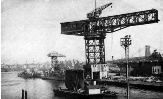
Work was also begun on construction of a new 350-ton hammerhead crane for installing turrets and guns aboard the new super-battle-ships. Caption: "Hammerhead crane in the Brooklyn Navy Yard" 1195
