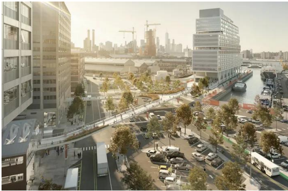
Caption: "With a new NYC Ferry landing opening in 2019, increasing connectivity between the dock, located in the back of the Navy Yard and the street (about a five-minute walk away) is a challenge. A new skybridge is proposed in the master plan." 1743
