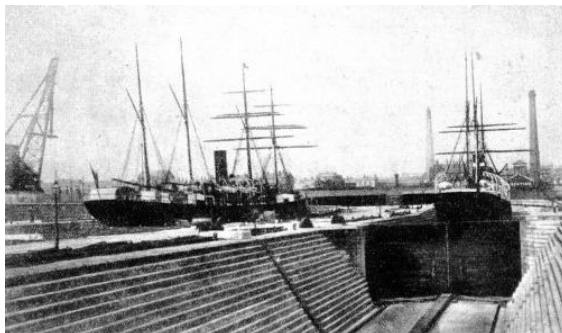
404 Caption: “OVER HALF A CENTURY AGO. Liverpool ship-repairing docks about 1883. At the present day there are twenty-one graving docks at Liverpool and Birkenhead. The largest of these, the famous Gladstone Graving Dock, was, at the time of its opening by King George V in July, 1913, the largest dry dock in Europe. The width at the entrance is 120 feet and the length 1,050 ft. 4 in.”
