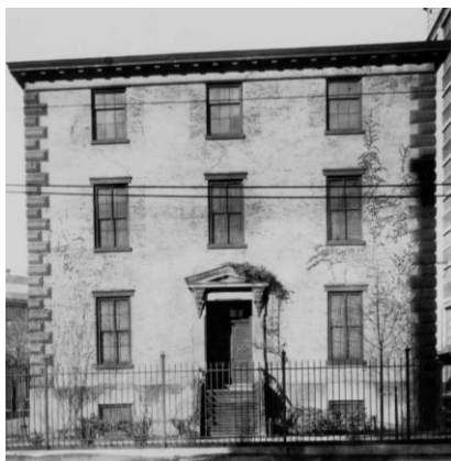
"...We proceed to a three-story landmarked building on Flushing Ave. designed by Thomas Walter, who designed the dome of the U.S. Capitol..." New York Daily News , July 28, 2011 Caption: "Building 92 South Elevation, 1932" 1613
