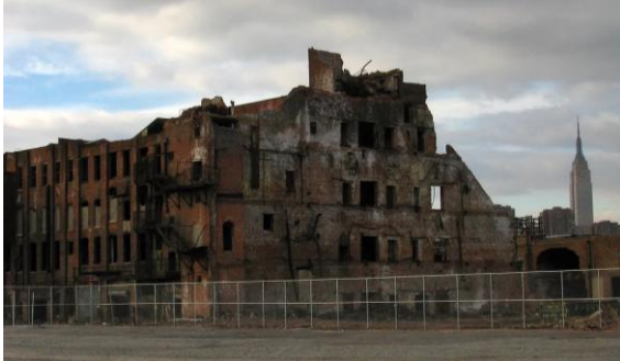
Caption: "The Greenpoint Terminal Warehouse, which burned in 2006, was largely demolished in 2007. 'If it wasn't a slow motion tragedy, it would be funny,' says Bankoff. 'Thinking about what the waterfront is going to look like 100 years from now, eventually we are going to have to build levees or some kind of protection against rising water, or just not have anything there.'" 1567
