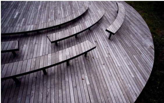
"...The surfaces of the walkway and entrance gateway are finished with black locust wood..." chi-athenaeum.org, 2017
