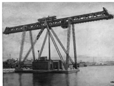
The structure consists of a steel pontoon which measures 100-feet in length by 60-feet in breadth and 11-feet 3-inches. Above the pontoon and parallel with its longitudinal axis is carried, at a height sufficient to give a lift of 45-feet and a reach of 45-feet beyond each edge of the pontoon, a pair of trusses which form the runway for a traveling crane trolley. The runway is carried upon massive latticed posts and struts, whose position and functions will be seen in our engraving.
