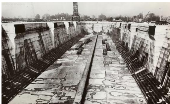
"...The dock, without a ship inside, contains 260,000 tons, or 58,000,000 gallons of water, and this can be pumped out in four hours..."
