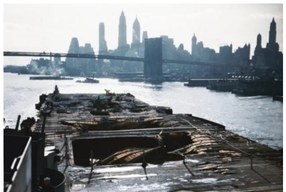
897 898 Caption: "USS Franklin , CV-13, on the East River, heading to the Brooklyn Navy Yard for repairs of bomb damage, 28 April 1945" 900
