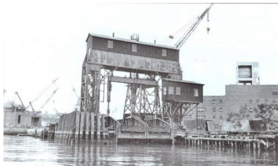
Above: the second Brooklyn Navy Yard float transfer bridge was installed ca. 1941, upon the completion of the Wallabout Basin expansion. It was an electrically powered overhead suspension “French Patent” type. This float bridge was modified in 1983, when the overhead supported dual spans (seen in the image above) were replaced with two pontoon supported float bridges. 292
