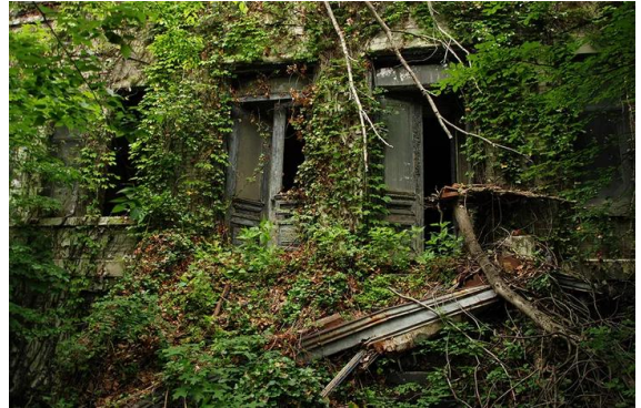
Caption: "The 11 residential buildings on the Admiral's Row campus have been completely overgrown by ivy and trees. The front steps of Quarters K and L are almost unrecognizable."
