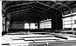
Above: caption: "Machine (right) and Shipfitter's Shops, St. Helena Area of the Norfolk Navy Yard. Note the welded steel sidings"
