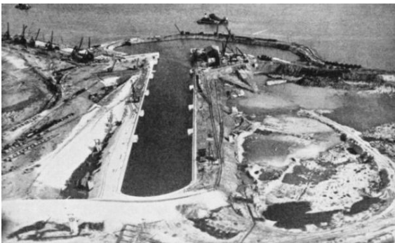
Caption: "BEHIND AN EARTHEN EMBANKMENT the reclaimed area was pumped dry and the huge graving dock built. When the dock was completed the embankment which covered the entrance to the dock was dredged away and the dock was open to the sea."
