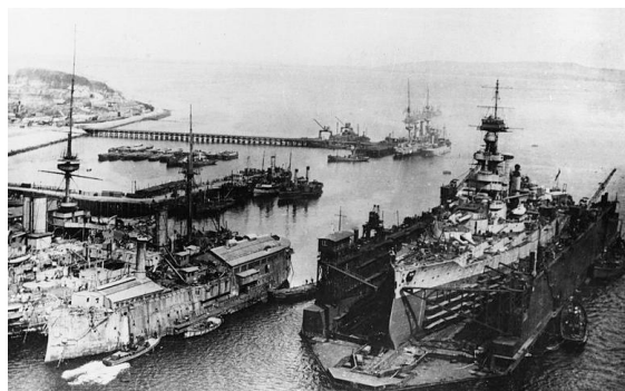
Caption: "The British battleship HMS Erin in a floating dry dock, ca. 1918. In the left foreground are several old warships employed as barracks."
