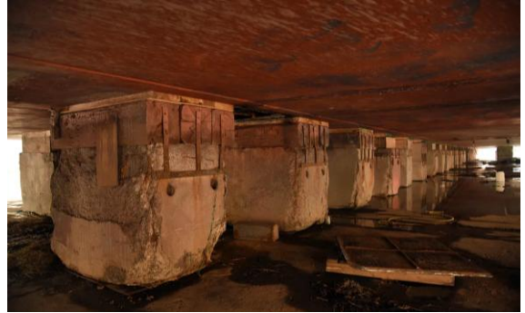
“...Down underneath this 11-story ship. ‘The blocks are concrete, and they have wood caps,’ explains Sanborn. ‘The wood caps are to protect the vessel, so it’s not just steel sitting on the concrete’...” ny.curbed.com, May 3, 2018
