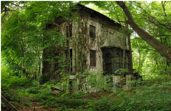
1545 Caption: "Building D, seen in 2015 before its demolition, was a charming three-story residence with wrought iron banisters and two attached sunrooms, surrounded by a lush forest"
