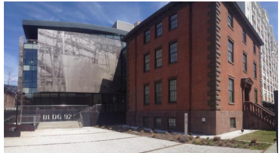
Above: closed in 1966 and dormant for decades, the 300-acre, 200 year-old Brooklyn Navy Yard has renewed life as an industrial park with sustainable design and construction as its operating principle. One of the premier projects was the "Brooklyn Navy Yard Center at Building 92," the adaptive reuse of and addition to the 1857 Marine Commandant's house, now housing a museum, leasable space for non-profit organizations and public amenities.
