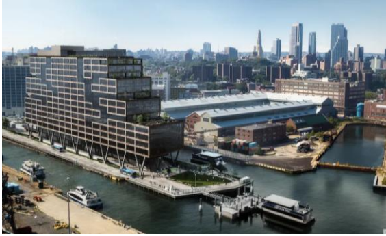
"...Built on an old dry dock, the building is raised above the floodplain, Patel said. In all, the building's design, he said, intends to express 'the old grid of Brooklyn Navy Yard in a modern way'..." ny.curbed.com, October 15, 2019
