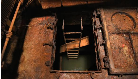
"...The lower depths of the caisson have been flooded with water to settle it into place. 'You could compare them to a sailboat, because they have a concrete bottom to keep them buoyant. Otherwise, they would just flip over,' says Sanborn..." 883 ny.curbed.com, May 3, 2018
