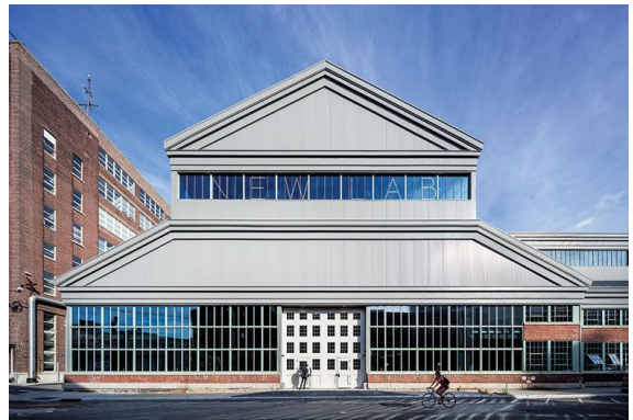
Caption: “Historically accurate insulated windows and cladding replace the existing envelope to bring the building up-to-date”
