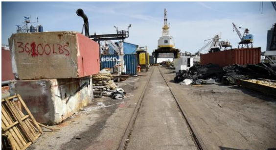
"...The docks of the shipyard are lined with a system of enormous cranes that have the capacity to lift 15 to 200 tons. The cranes can be used to lower the dry dock blocks down into the graving docks. These concrete blocks weigh three to five tons, and are used to support ships when water is pumped out of the dry dock..." 885 ny.curbed.com, May 3, 2018
