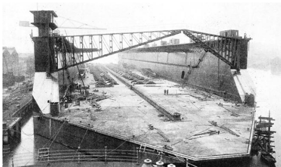
Caption: “WORLD’S LARGEST FLOATING DOCK in the final stages of completion. Built in 1922 by Armstrong, Whitworth, for the Southern Railway, the Southampton floating dock has a lifting capacity of 60,000 tons. It is 960-feet-long, with an overall width of 170 feet and a clear width inside of 130 ft. 6 in. The total floor area of the dock is about 3½ acres.”
