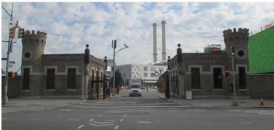
Above: the Sand Street Gatehouse has undergone modifications throughout the years, including the addition of second and third floors (since removed) and the removal of the turrets. After the Brooklyn Navy Yard was decommissioned in 1966, the Sands Street Gate became the entrance to the NYPD’s Brooklyn tow pound and by 2004, there were plans to refurbish the gate. The gatehouse was restored to its original condition in 2012 and since 2015, it has housed the Kings County Distillery’s tasting room.
