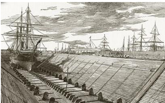
Above: the dry dock at the Erie Basin was a type of Simpson Dry Dock Co. timber dry dock that James E. Simpson patented in 1854
