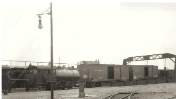
Also located on the Marine Channel were four freight piers operated by various railroads and a municipal refuse pier. The Marine Channel was separated from the yard basin by a causeway of heavy masonry construction which connected the Cob Dock area with the main yard. Two cruiser piers projected into the yard basin from the causeway. 293
