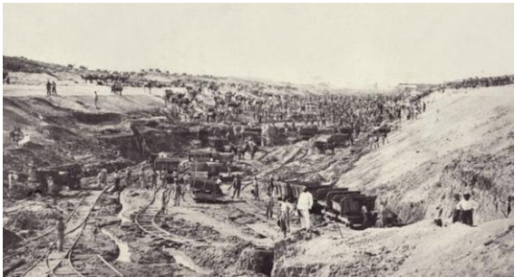
Caption: "Digging by hand, a huge work gang excavates a sandy stretch of the canal amidst a tangle of dumpcart tracks, while camels, used for bringing food, drink and equipment, browse on the skyline. In marshy places, workers had to stand waist-deep in water, scoop-up the mud with bare hands and squeeze it dry against their chests before depositing it on the banks."
