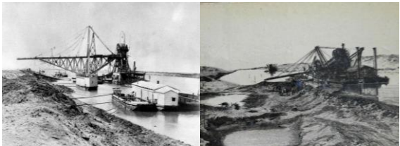
"...When the channel was sufficiently deep, dredgers were floated in to remove the soil more quickly, the soil being cleared from the channel by means of a contrivance similar to a great iron sp-out. It was 230-feet-long, 5-1/2-feet-wide, and 2-feet-deep. The soil was dumped into it, converted into sludge by water, and then pumped clear of the channel..." Shipping Wonders of the World , ca. 1937 Left: caption: "Dredging work being carried out on the Suez Canal prior to its official opening in 1869" Right: caption: "Dredger operating near the Bitter Lakes"
