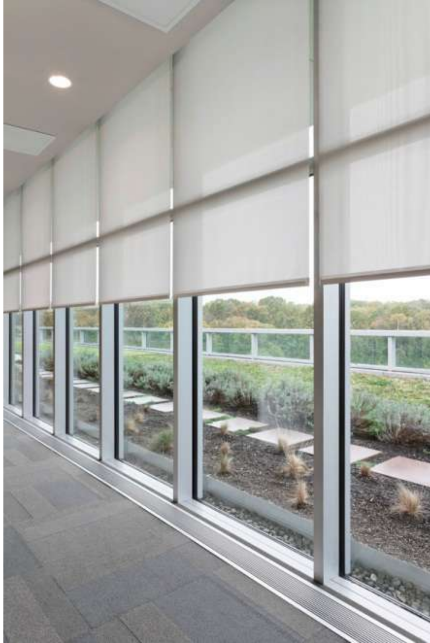
Figure 17 Example of Solar-Adaptive Shading
