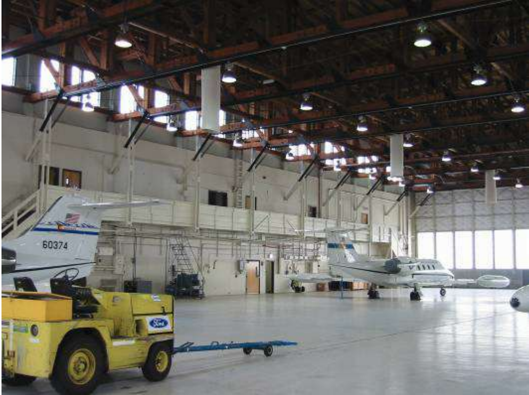
Figure 12 Example of Clerestory Application
