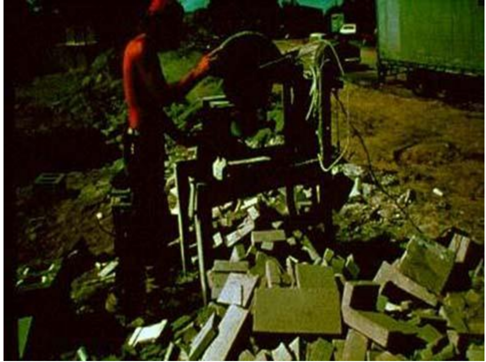
Figure 12. Worker cutting material with saw.
