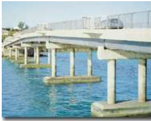
Tropical Marine: Bridge by the Ocean
