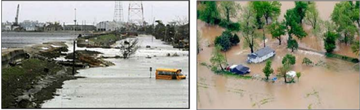
Photos - Levee Failures in New Orleans and Missouri
