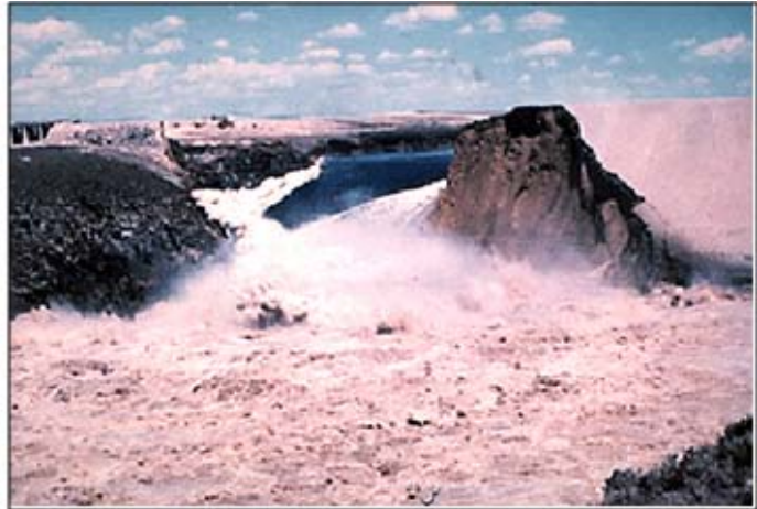
Photos - The Failure of Teton Dam, June 5, 1976
