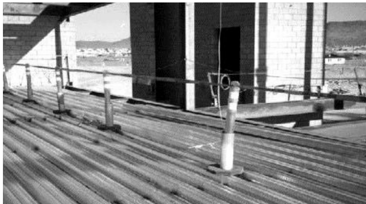
Controlled decking zone
