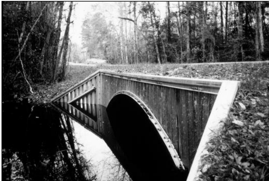
Figure VI-36--Long Span Culvert (Contech)
