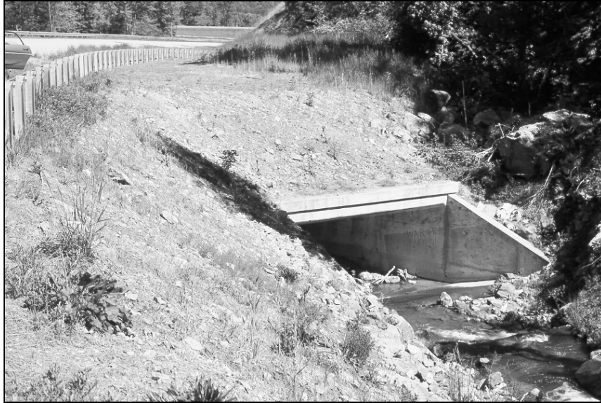
Figure VI-20--Fill Warped to Avoid Inlet Skew
