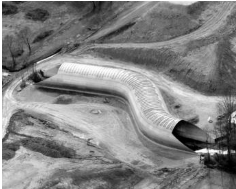
Figure VI-4--Culvert with a Horizontal Bend (Contech)
