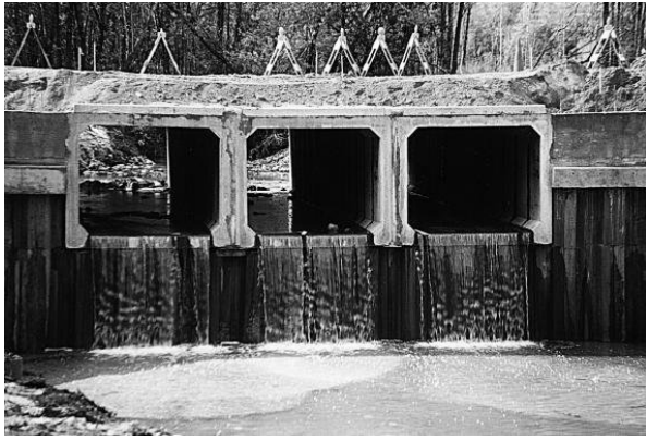
Figure I-5--Precast Concrete Box Culvert (American Concrete Pipe Association)
