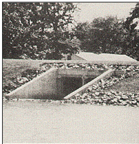
Figure VI-1--Stormwater Management Pond with Culvert as Outflow Control Device
