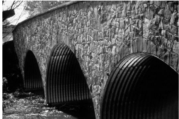
Figure I-6--Corrugated Metal Arch (Contech)
