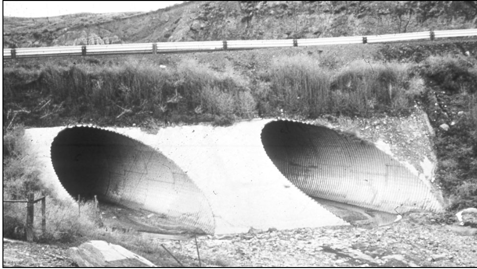
Figure VI-34--Slope Paving Around a Mitered Inlet
