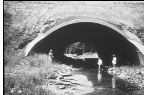
Figure I-2--Long Span Culvert
