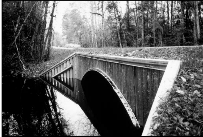
Figure VI-10--Culvert with Metal Headwall and Wingwalls (Contech)
