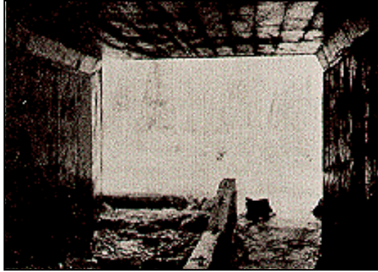
Figure VI-7--Fish Baffles in Culvert
