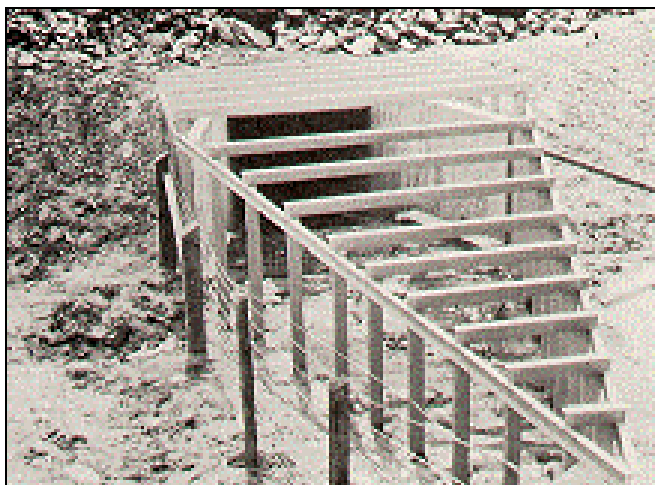
Figure VI-16--Debris Deflector
