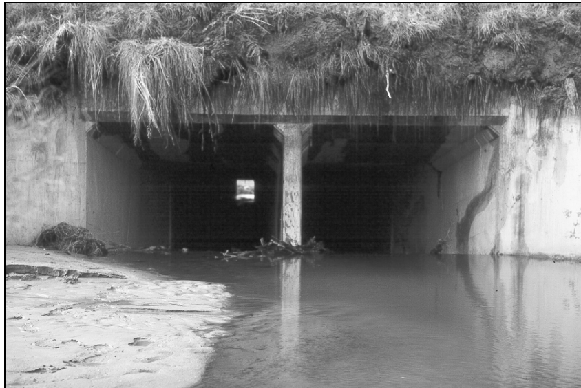
Figure VI-21--Double Barrel Box Culvert
