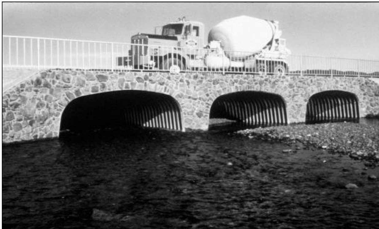
Figure VI-24--Corrugated Metal Box Culvert (Contech)
