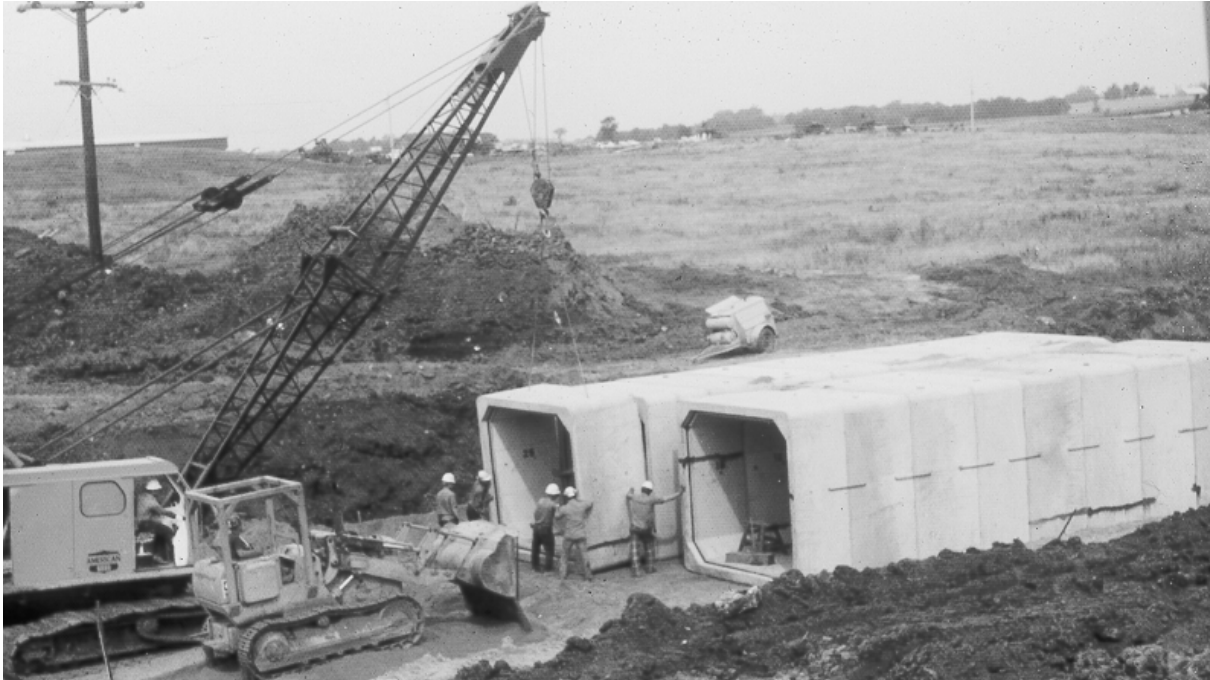
Figure VI-25--Precast Double Barrel Box Culvert
