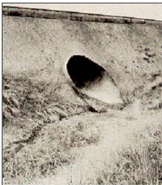
Figure VI-33--Unanchored Mitered End
