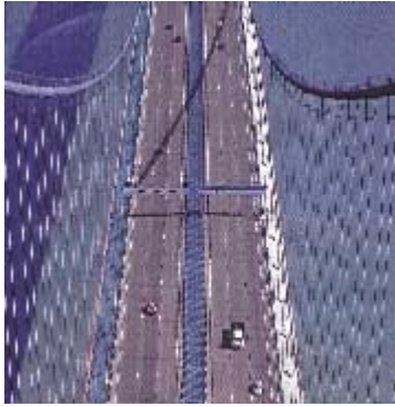
Figure 14: Aerial view of part of the Tsing Ma Bridge, Hong Kong.
