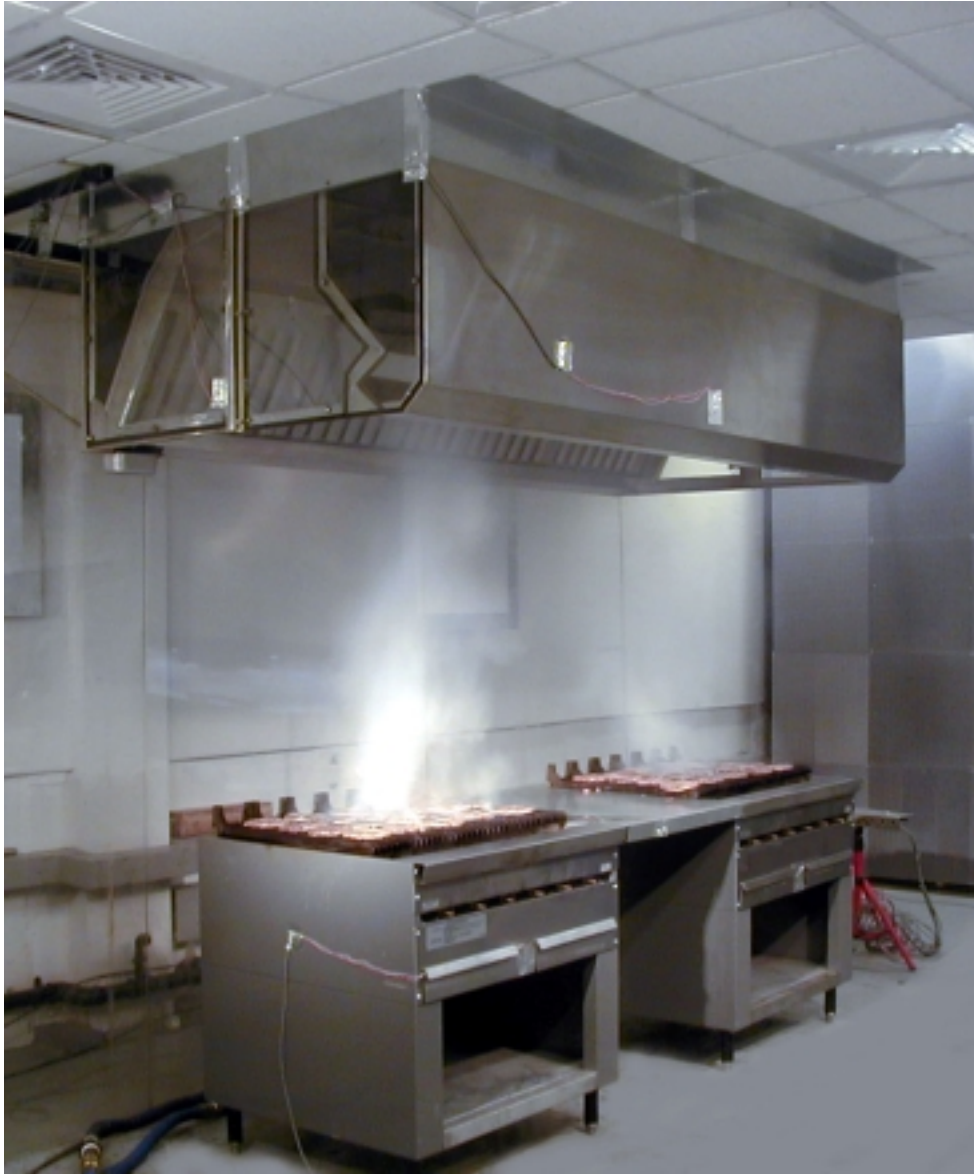
Figure 10: Cooking Test of Two Gas Charbroilers under a Wall Mounted Short Circuit Canopy Hood
