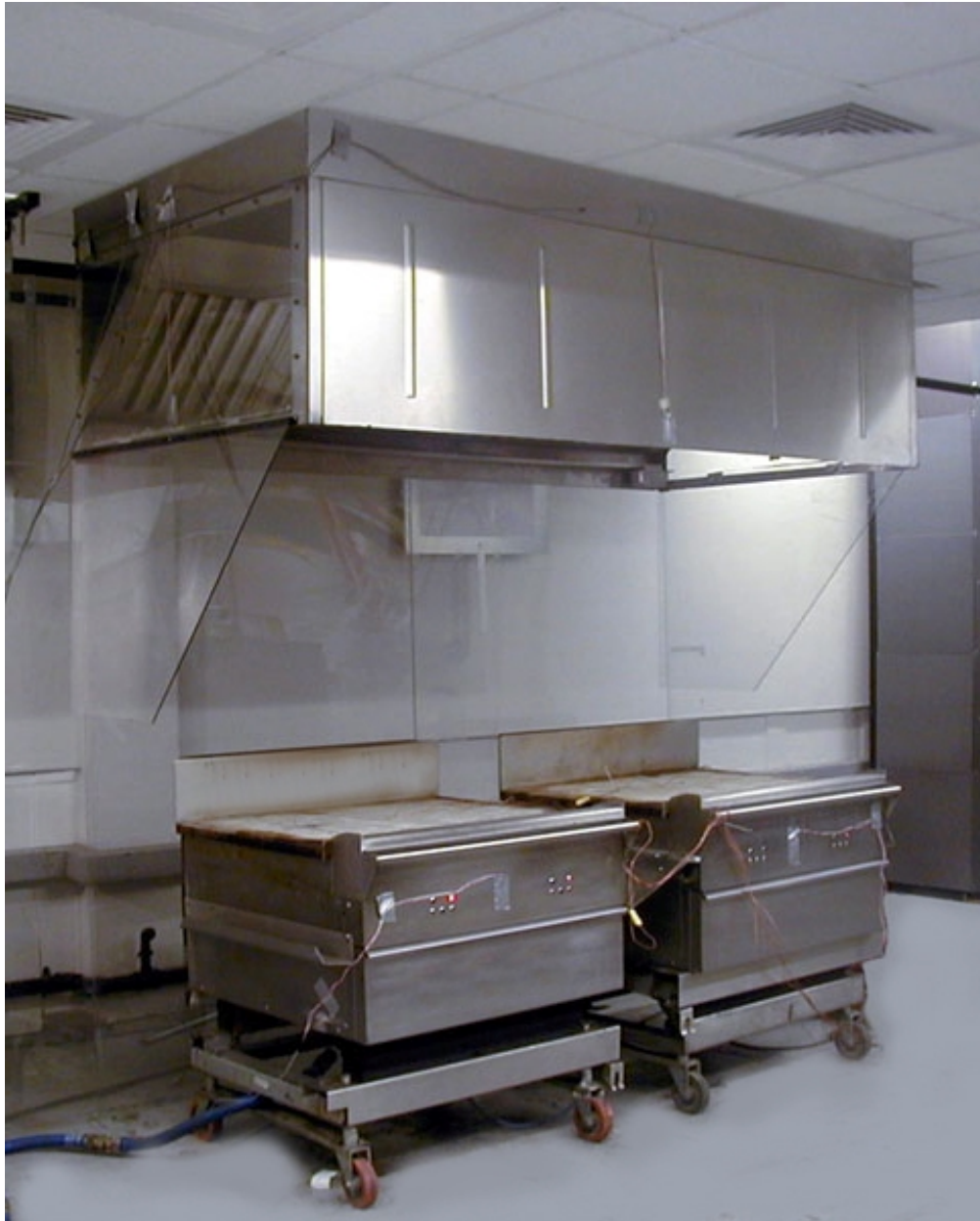
Figure 6: Two Griddles Under an 8' Exhaust Hood with Transparent 1/4 Side Panels
