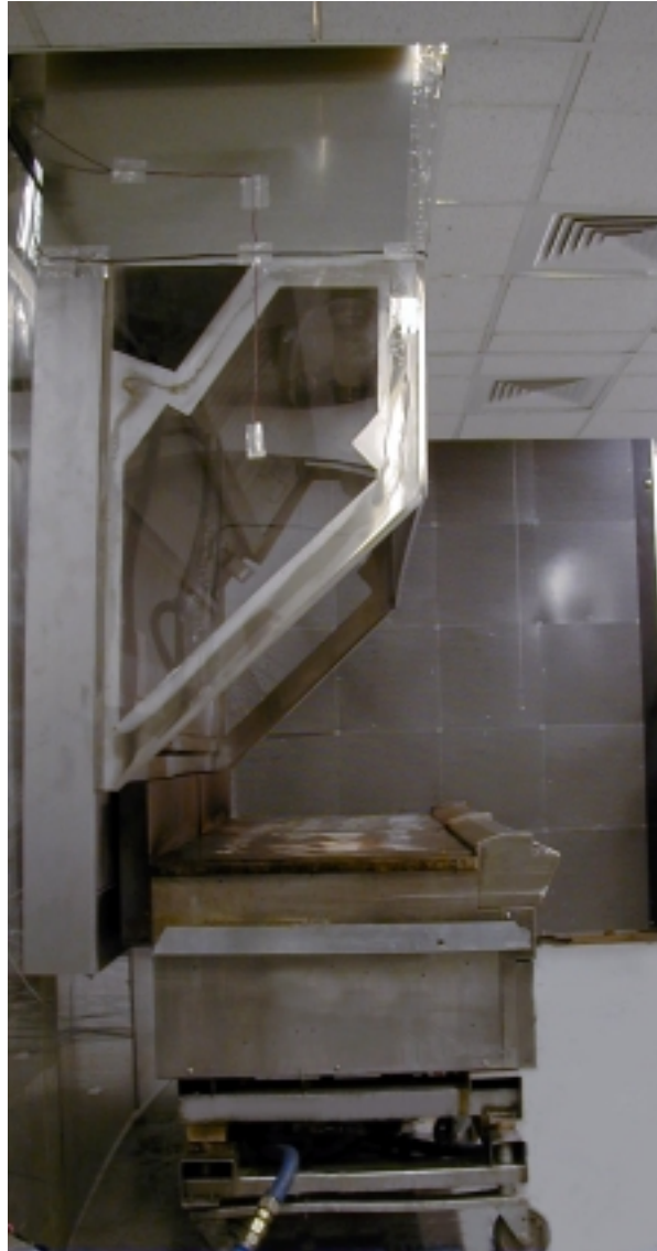
Figure 84: View of Two Griddles under a Backwall Supply Proximity Hood from the Perspective of the Schlieren Visualization System
