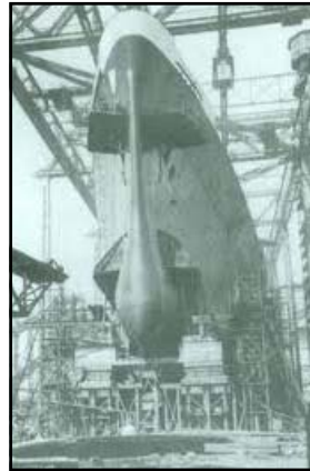
"...The ship's bow presents a number of unique and promising characteristics. It is neither like the full bulbous bow on the Bremen (at left) nor like the old fashioned knife-edge type, but is clipper shaped with a very graceful semi-bulbous effect near the keel; it curves up into a rounded, streamlined rigid deck covering such as no ship is known to have..." Popular Mechanics, Dec. 1932
