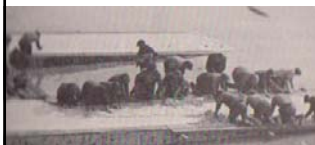
"...Planning the launching way is the first step in building a vessel. A double track of wood, leading to the water's edge and extending a short distance beneath the surface – called the 'standing ways' – serves as a runway for a pair of cradles known with their platforms as 'sliding ways.' These support the vessel's bow and stern during launching..." Popular Science , February 1933
