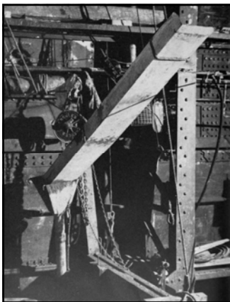
Tremie concrete pipe rig
