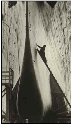
Normandie's "Protruding Forefoot" (a.k.a. Protruding "Bulb" or "Nose") The shape practically eliminated the bow wave and left a flat wake astern of the ship, greatly increasing hydrodynamic efficiency.
