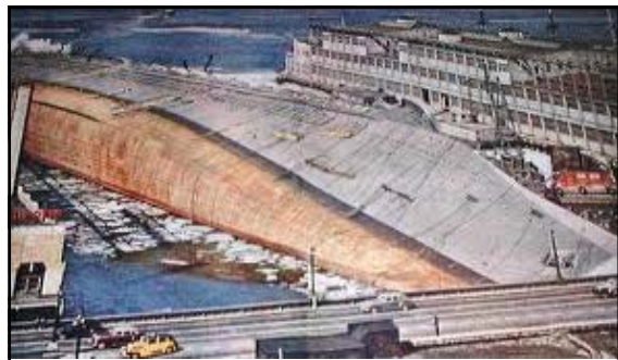
View of hull (from nearby building – elevated West Side Highway in foreground)
