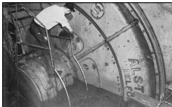
Starboard Inboard Engine (partially submerged) (both port engines were completely submerged)
