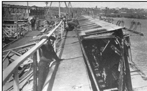
Removing structure above Promenade Deck
