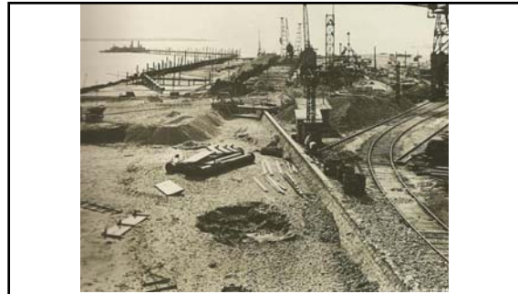
New dry dock "Number One" under construction at the Penhoet shipyard in St. Nazaire – built specifically for Normandie . The work began in October 1929 and was completed a few weeks before Normandie 's launch in October 1932.
