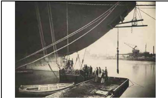
Rudder Installation November 1933
