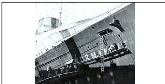
Removing her name from the bow. Normandie's expeditious conversion to a troopship took place at her Pier 88 berth. As a troopship (designated AP-53), she could carry 18K troops at one time (about 338K each year of the war). On her upper decks, fourteen 50mm anti-aircraft guns were installed on newly added platforms. On three of her lower decks, steel plates were welded over all porthole openings. 626
