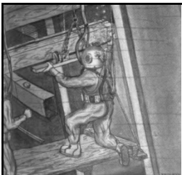
Above: timber and cradle used to lower bulkhead timbers to the divers
