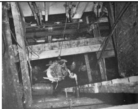
Hoisting rubble through open cargo door
