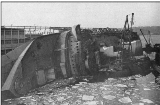
Removal of stacks
