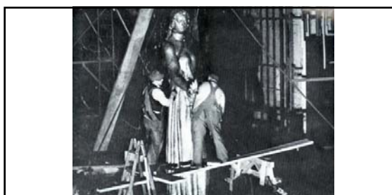
The eighteen-foot tall gilt bronze sculpture by Louis Dejean of a peasant woman of Normandy province (placed in the middle of the Main Dining Room ) is carefully prepared for removal. During the conversion, Normandie was stripped of her artwork and interior fittings in preparation for service as a troopship. Anything "fancy" had to go including the glass panels on the walls of the Grand Salon , the Lalique crystal chandeliers and fixtures in the Main Dining Room etc. Only the Sun Deck Suites would remain intact (for high-ranking officer's use). 628
