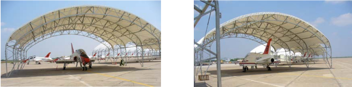
Figure 6-7 Examples of Weather Covering
