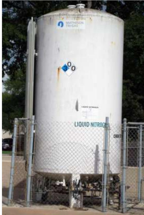
**FIGURE 13: VERTICLE STORAGE TANK FOR LIQUID NITROGEN**
