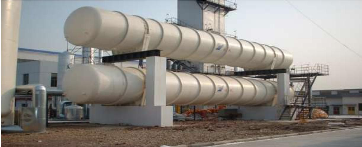
**FIGURE 15: HORIZONTAL CRYO STORAGE TANK SYSTEMS****PIPING AND TRANSFER OF CRYOGENIC LIQUIDS:**
