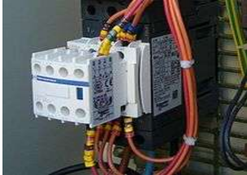
AC Contactor for a circuit application:
