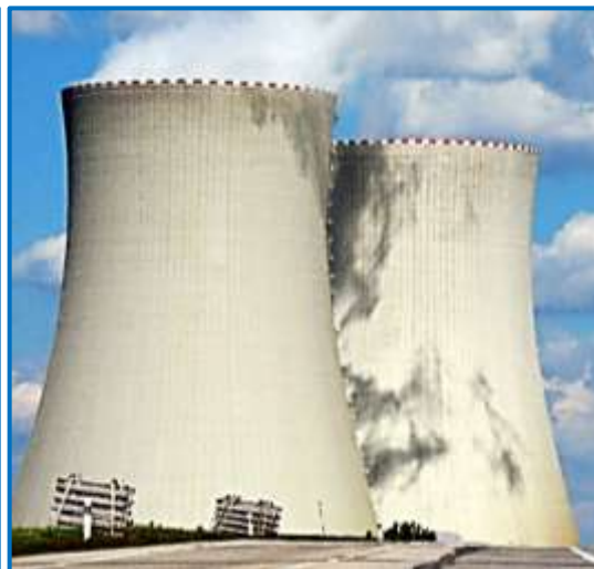
Natural Draft Towers
