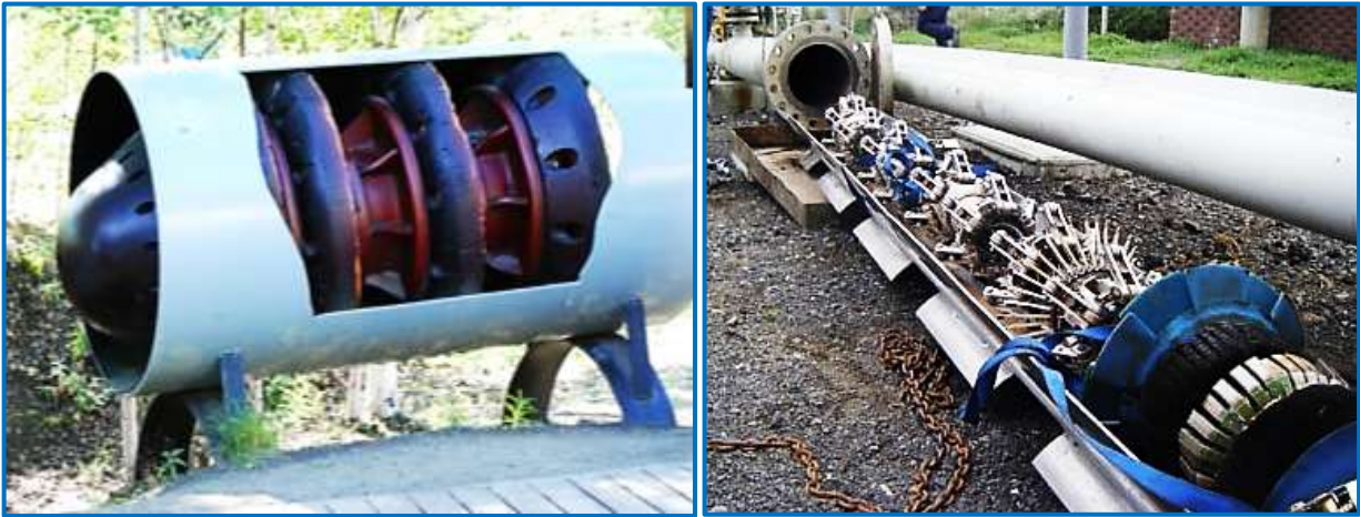
Pipeline inspection with “pigs”
