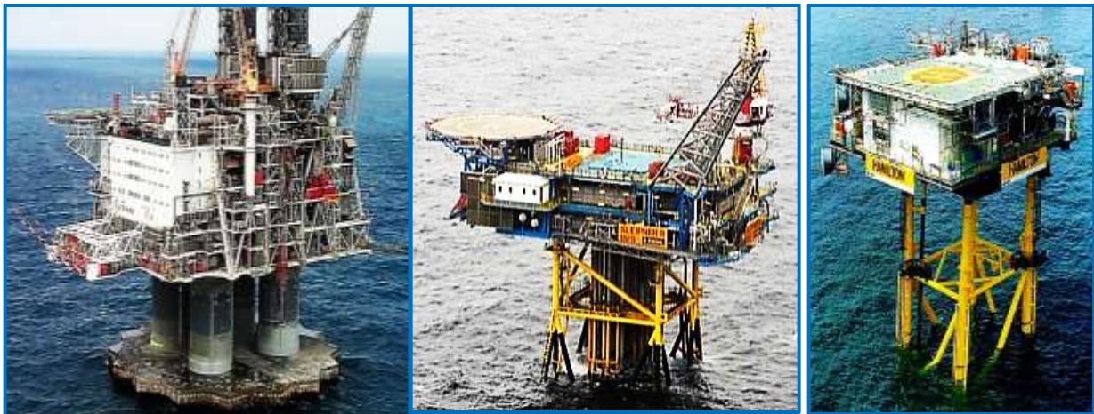
Gravity-Based Structure– GBS - Normally Unmanned Installations (NUI) - Satellite Platforms
