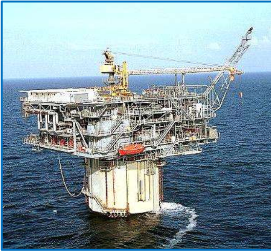
Floating Spar Platform
