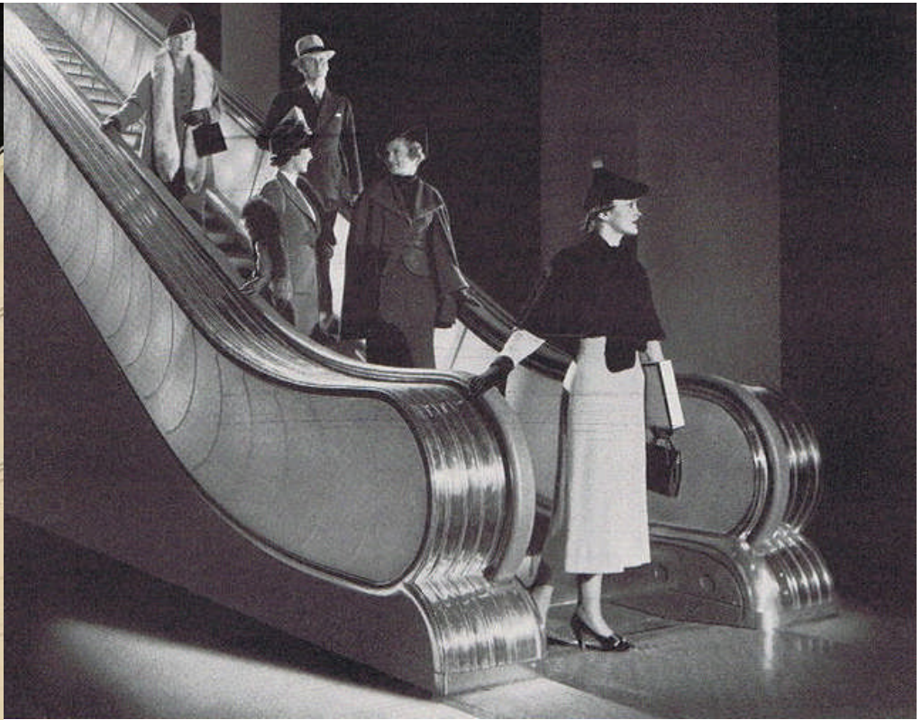
Above: caption: “Interior and exterior balustrading of The Emporium Escalators is of a sand-blasted glass, coral tinted in some places. It is illuminated from within, and nickel-bronze metal is used for accent.” (from a 1936 Otis ad)
