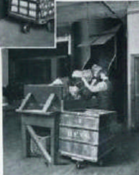
Outlet of Spiral "C" at 6th floor.
