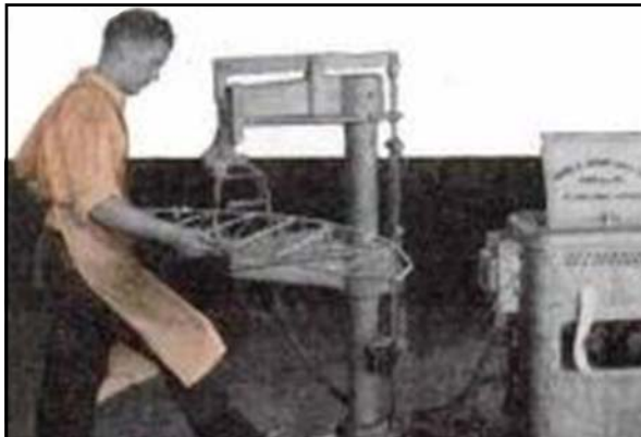
Caption: "Shot-weld apparatus, and tape on which are recorded the heat units in each weld" 565
