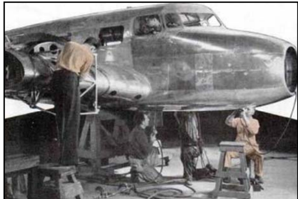
Caption: "Building the first all-metal transport – the 200-mile-an-hour Lockheed Electra. Here we see workmen busy on nose and wing."
