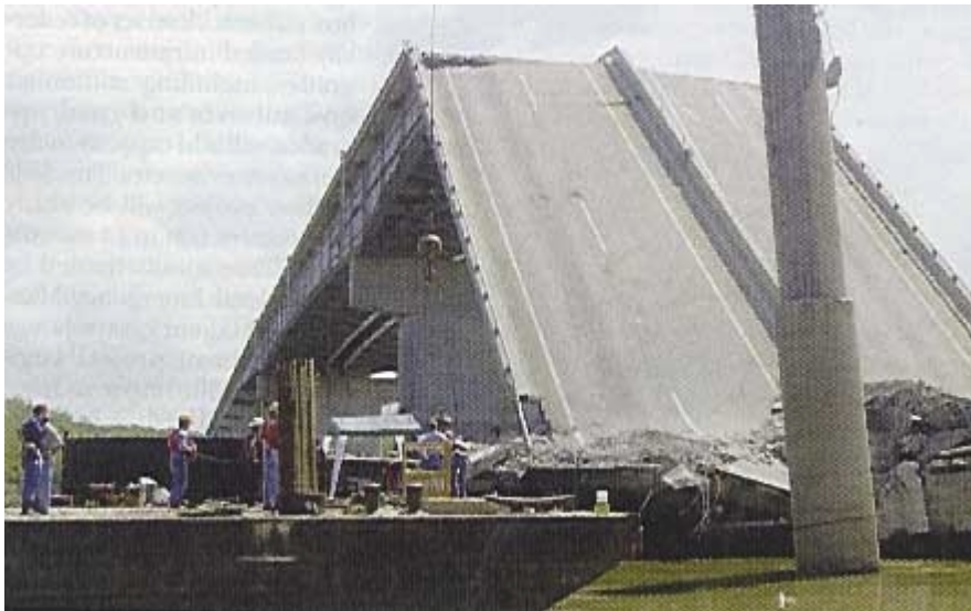
Figure 8: The barge in the foreground shattered bridge piers causing a section of the interstate highway to tilt into the river.
