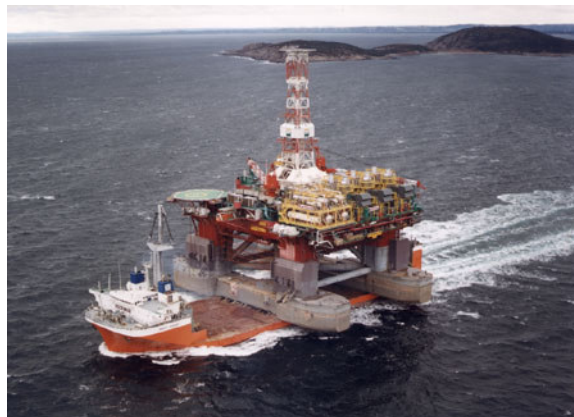
Figure 7.4: The Petrobras P-36 oil platform.
