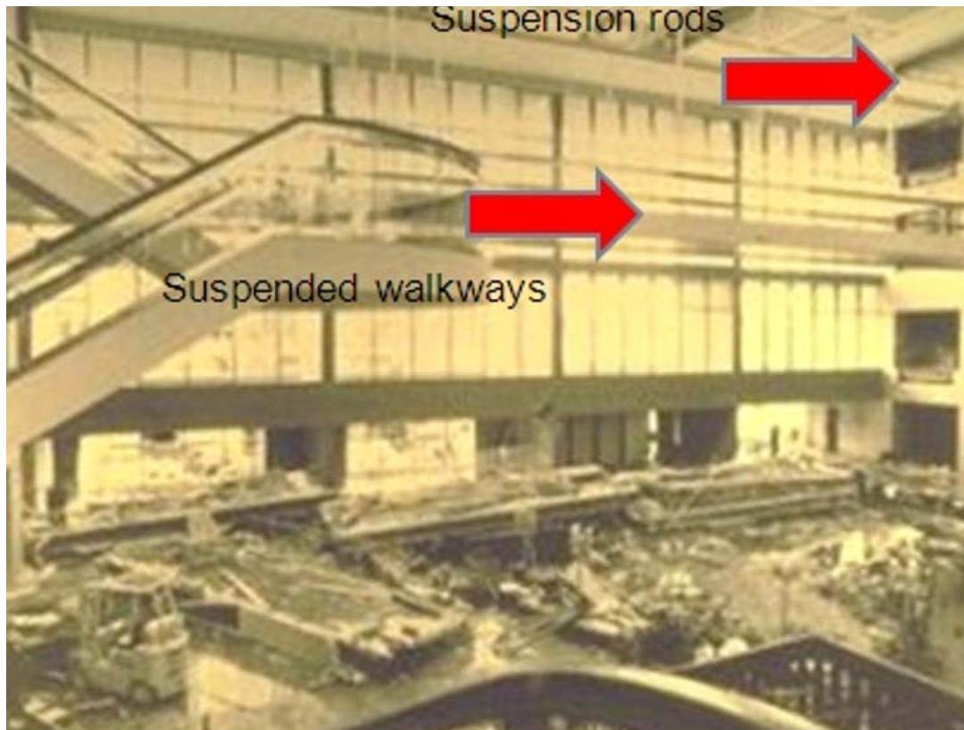
Figure 5 Suspended Walkways at the Atrium Lobby
