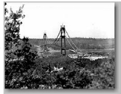
Tacoma Narrows Bridge Under Construction (University of Washington Libraries, Special Collections, PI-20789)
