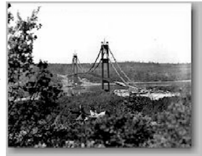
Tacoma Narrows Bridge Under Construction (University of Washington Libraries, Special Collections, PI-20789)
