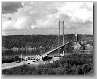
Tacoma Narrows Bridge Completed (University of Washington Libraries, Special Collections Division, PH Coll. 290.24)
