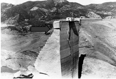
St. Francis Dam, March 17, 1928 (Attribution: U.S. Geological Survey Photographic Library)
