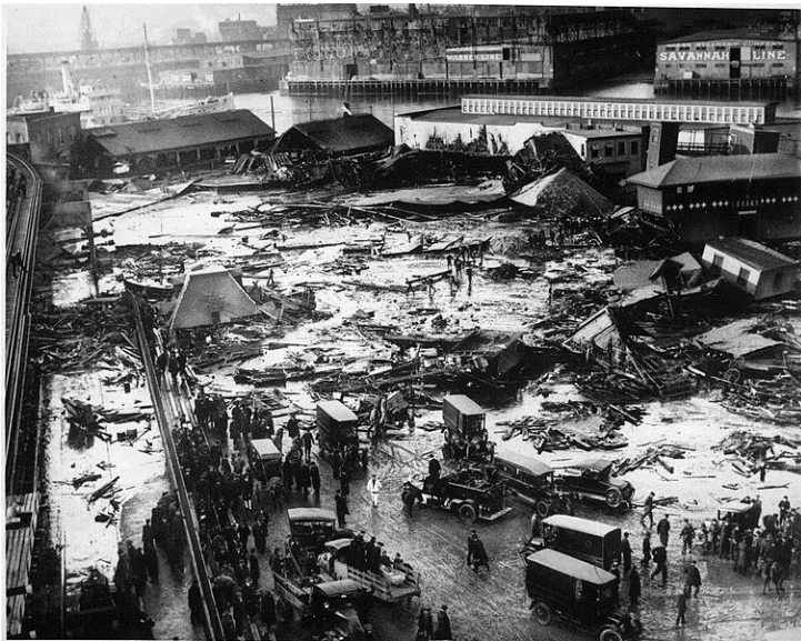
Figure 1. Aftermath of molasses tank failure
