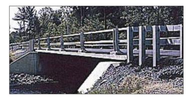
Weathering Steel can be as readily painted or coated as regular carbon steel. In its unweathered condition, a good wire brushing and solvent washdown is adequate to remove loose material, dirt and other contaminants before painting with a chromate oil-based paint. For synthetic resin paint (vinyl, epoxy, acrylic or alkyd) and inorganic zinc systems, blast cleaning or the equivalent is suggested.
