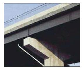
Another factor important to the success of Weathering Steel structures is the elimination of any details that prevent normal wet-dry cycles. The retention of water, dirt and other debris must be avoided and natural drainage should be designed into the structure. Tubular and box sections should be sealed or adequately vented to allow air circulation, prevent condensation and allow for drainage.
